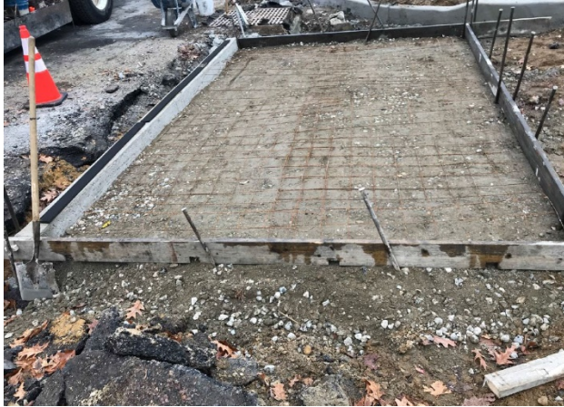
Figure 4: Driveway reinforcement
