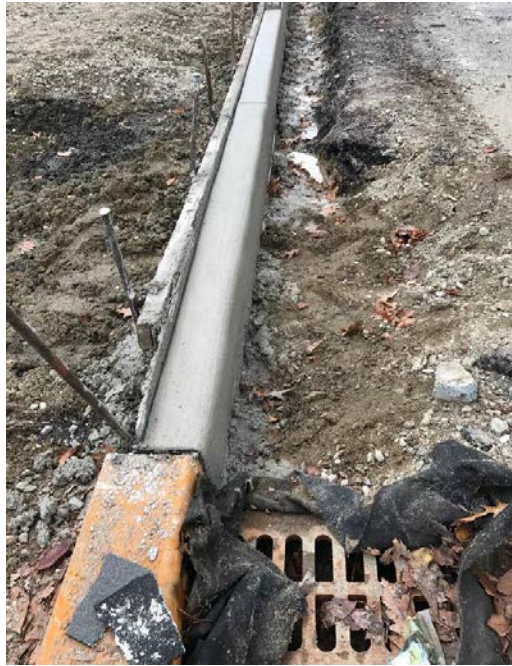
Figure 1: Concrete curb
