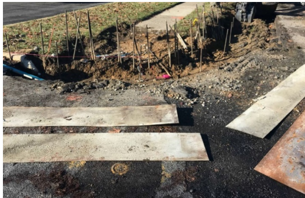
Figure 2: Concrete curb ramp forms
