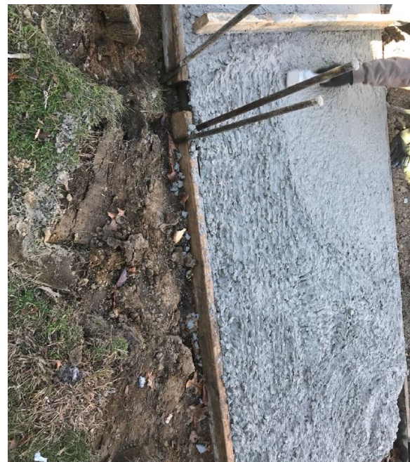
Figure 3: Concrete sidewalk placed
