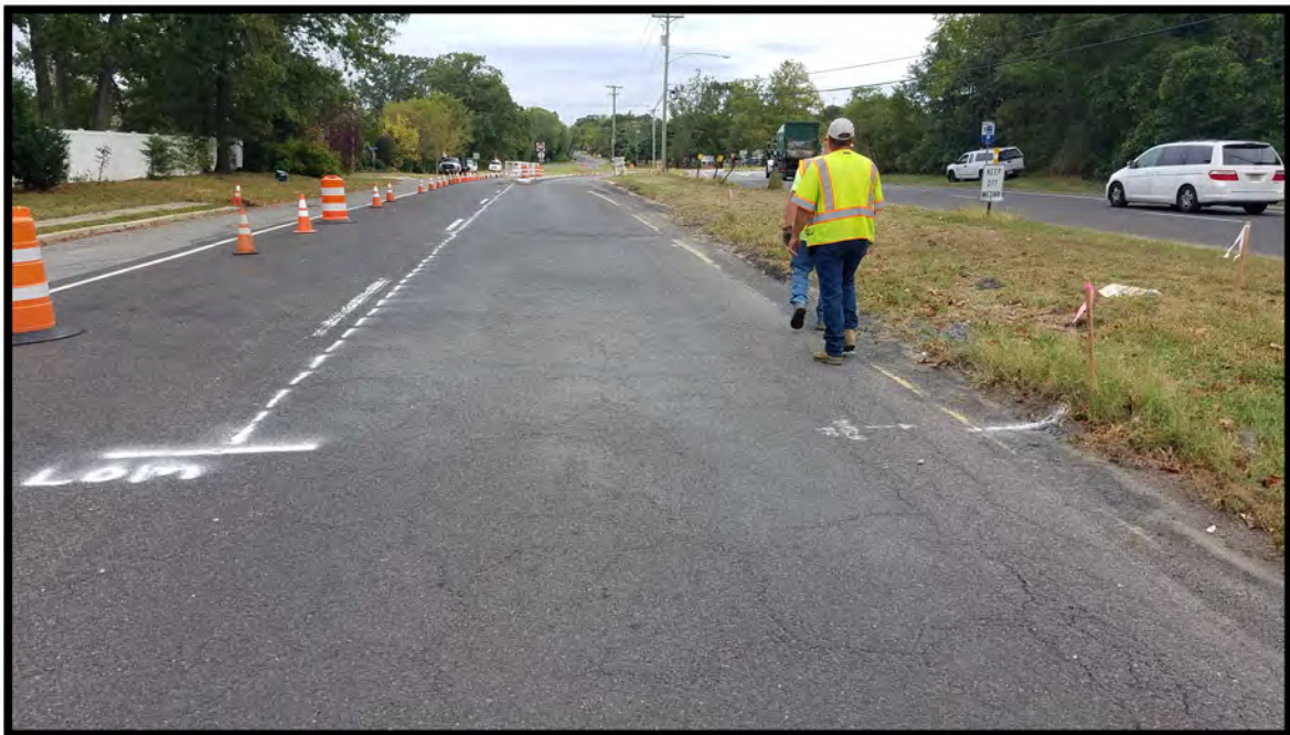
10. Laying out mill and overlay limits.
