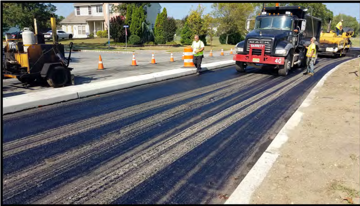
11. Roadway milled, tacked and elastomeric joint adhesive installed adjacent to curb.
