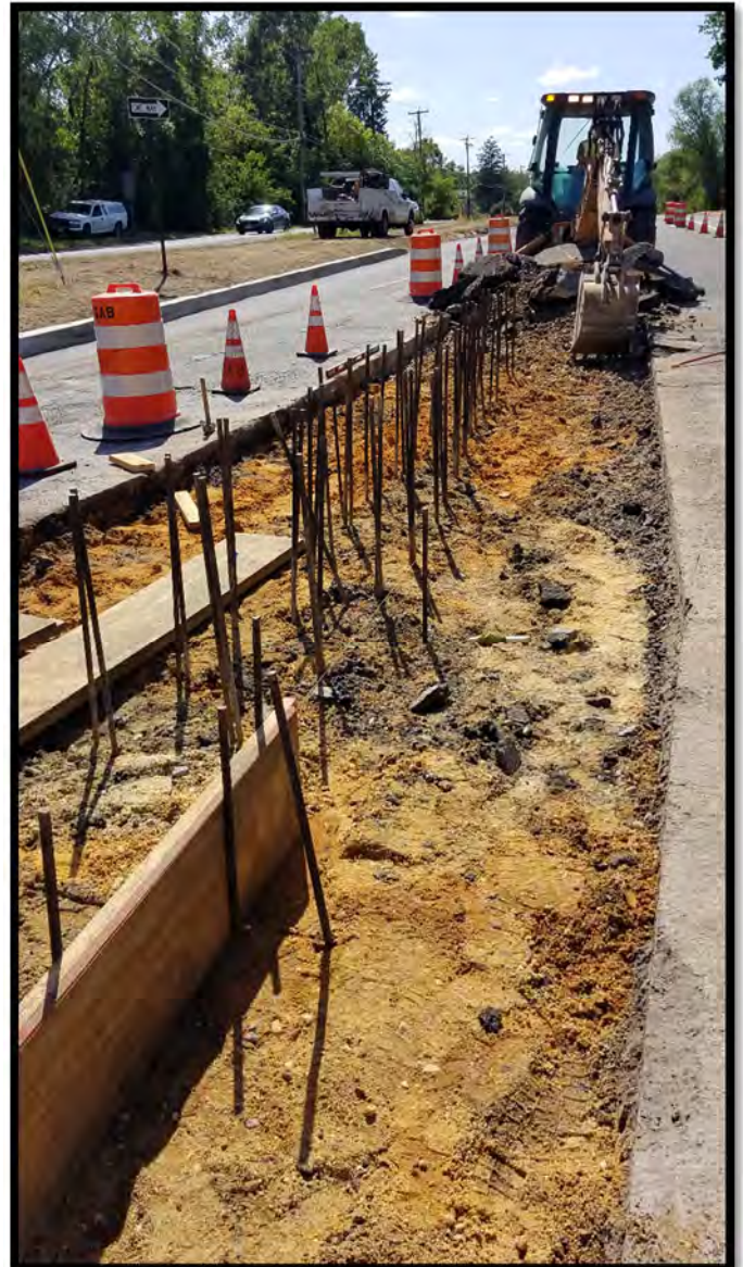
6. Curb forms being installed for extended concrete island.
