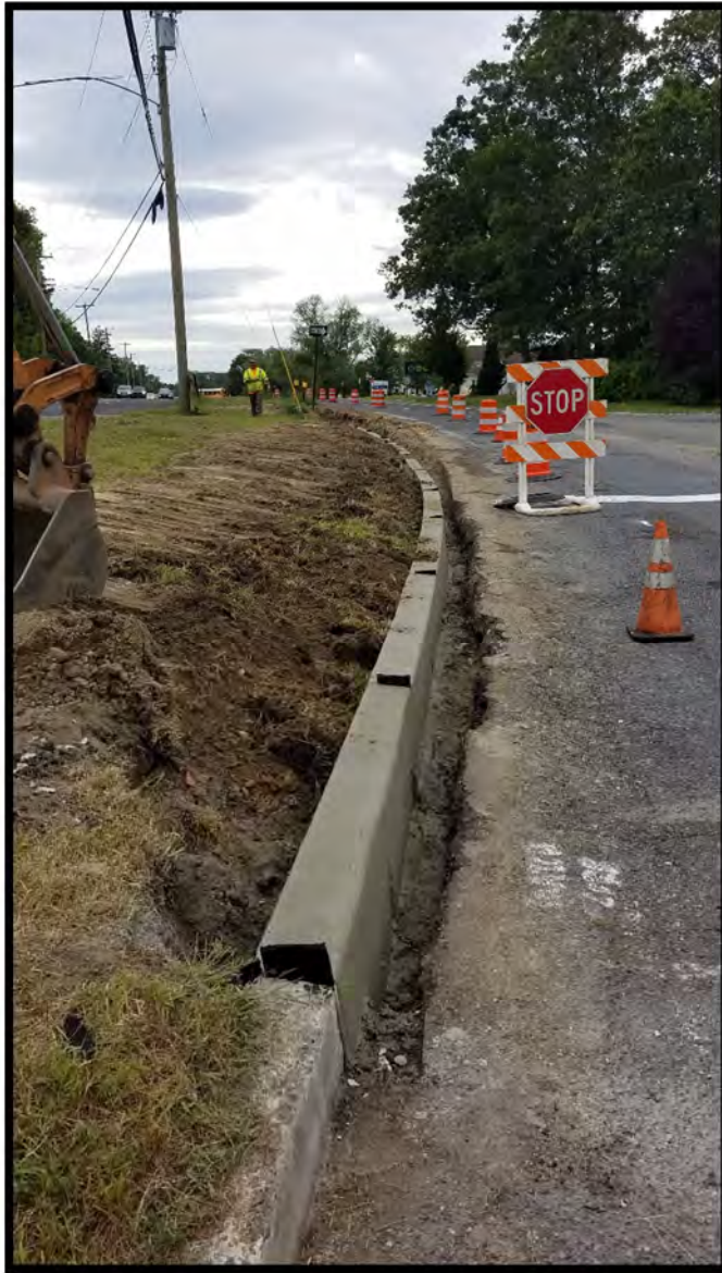
1. New curb installed at widened ramp lane.
