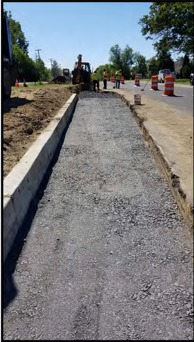
3. Compacted Dense Graded Aggregate at widened ramp area.
