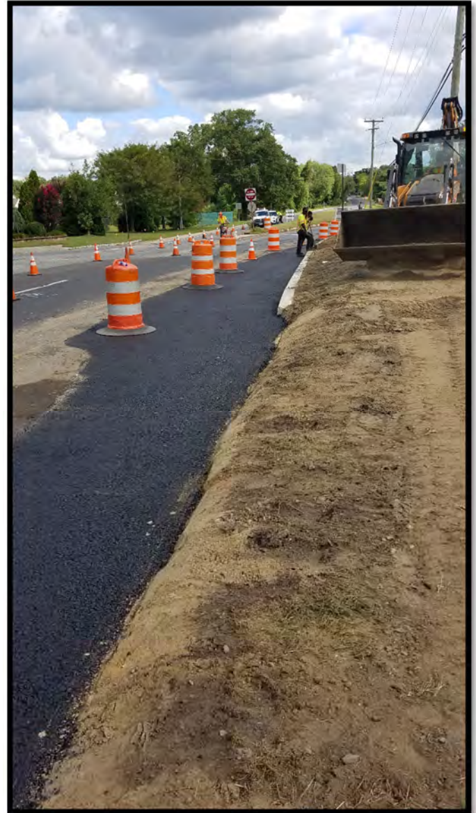
4. Hot Mix Asphalt installed at widened ramp area.
