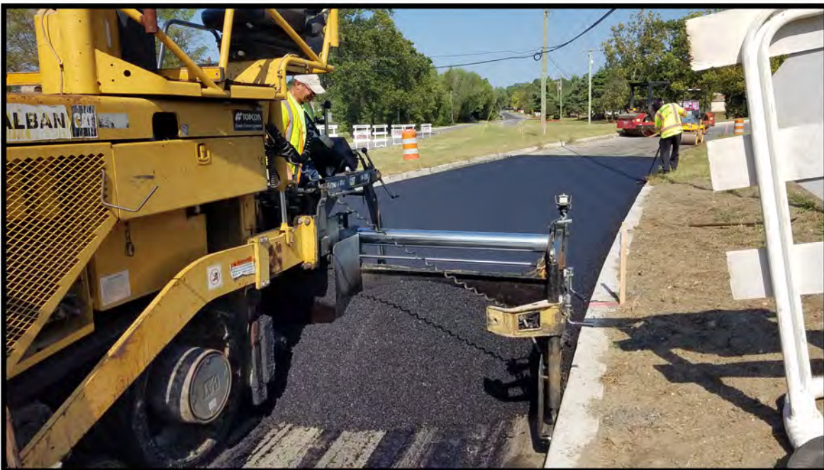
12. Hot Mix Asphalt overlay being installed.
