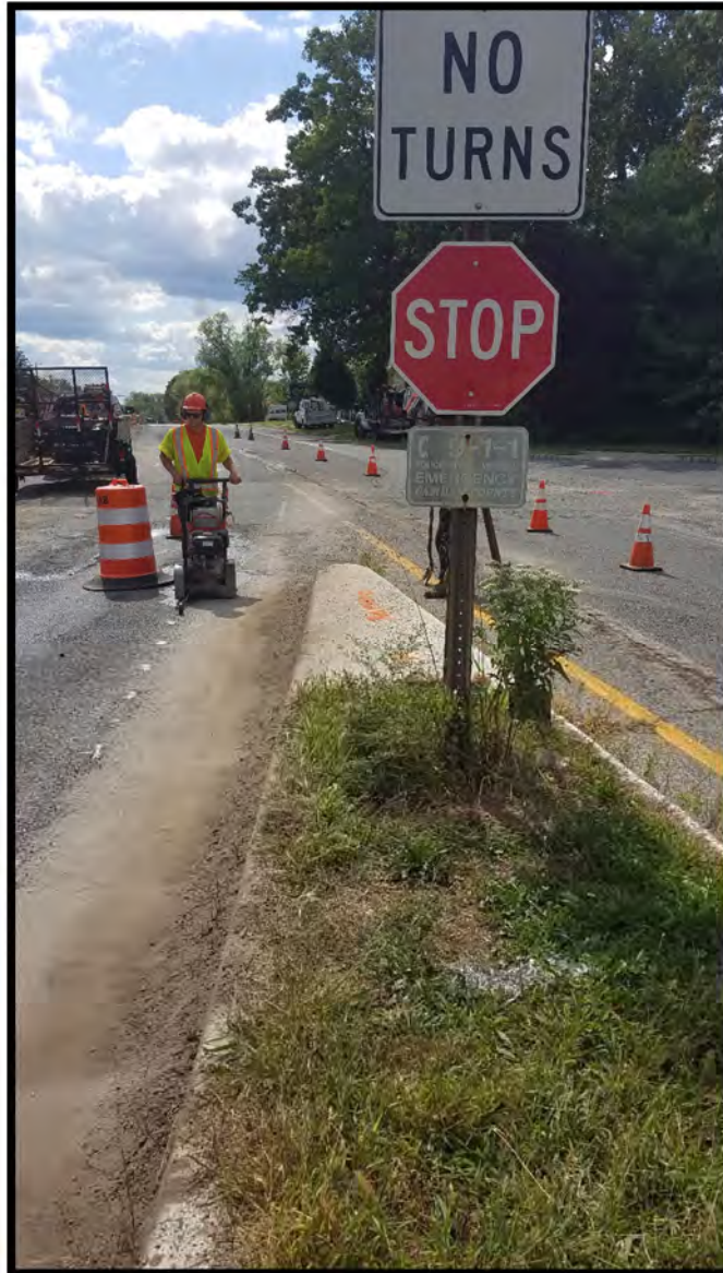
5. Sawcutting to install new curb at extended concrete island.
