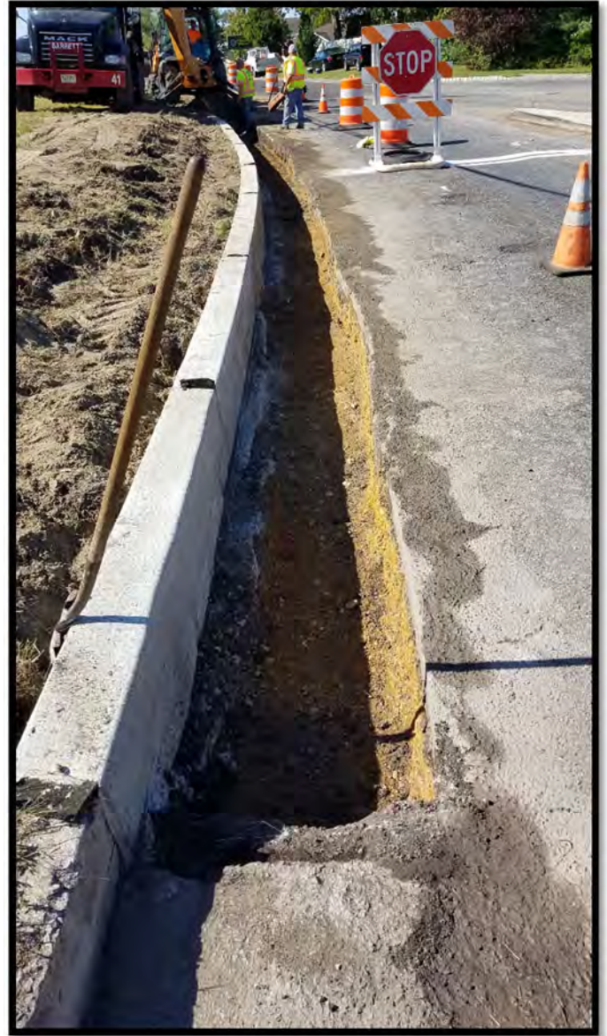
2. Boxing out for pavement restoration adjacent to new curb.
