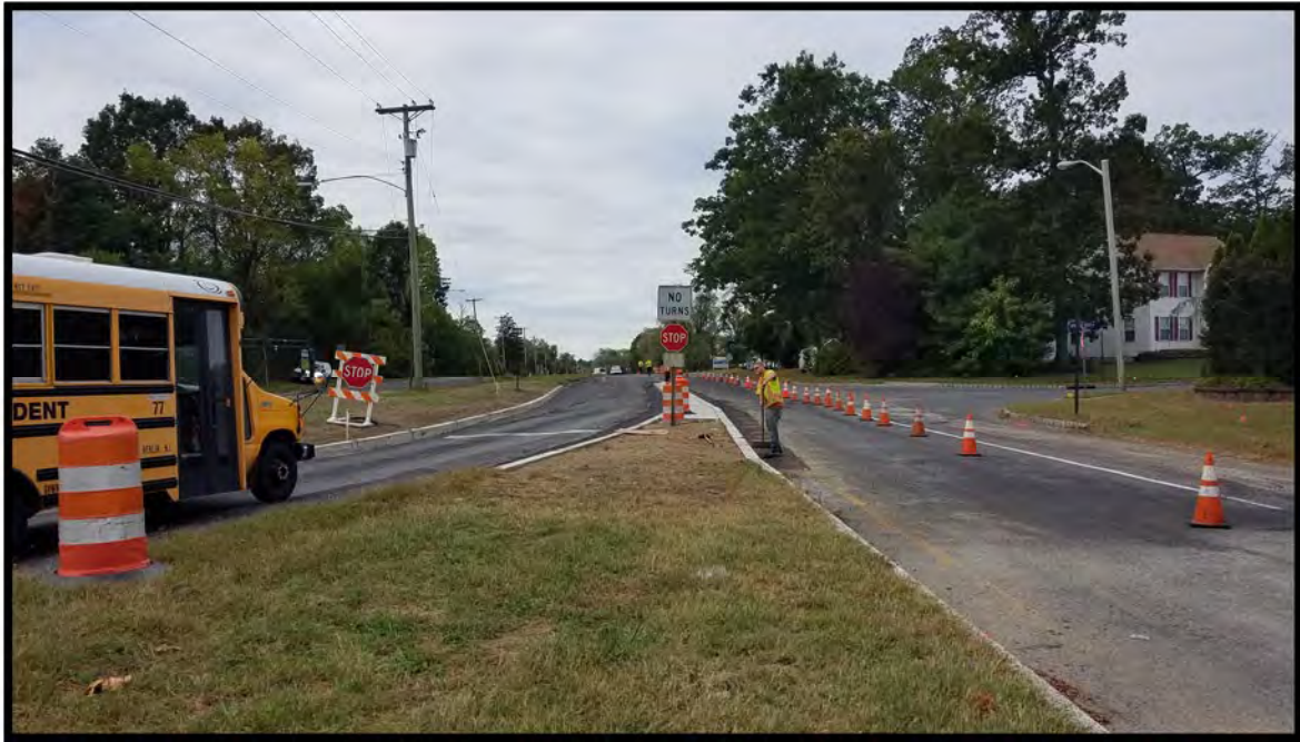
9. Concrete flatwork complete and preparing for mill and overlay.
