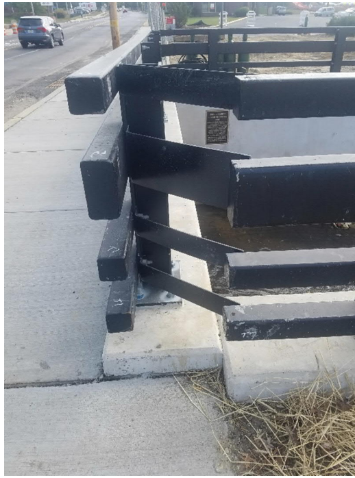
Safety bars installed on bridge railings
