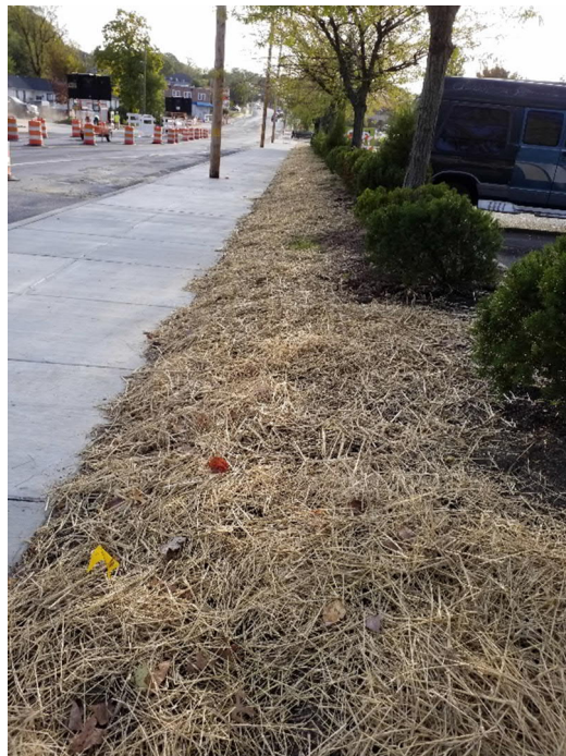
Topsoil, fertilizer, seed and straw placed
