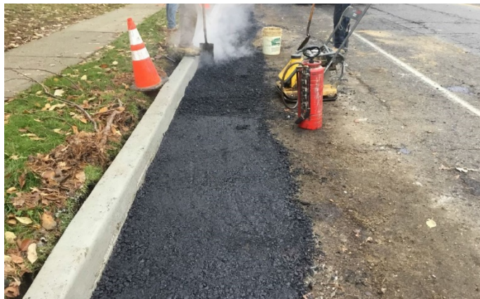
Figure 2: Asphalt restoration
