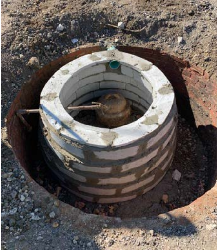
Figure 2: Manhole reconstruction
