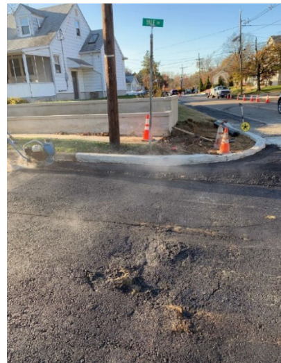
Figure 5: Reconstructed roadway section
