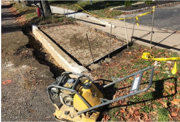
Figure 4: Concrete driveway reinforcement
