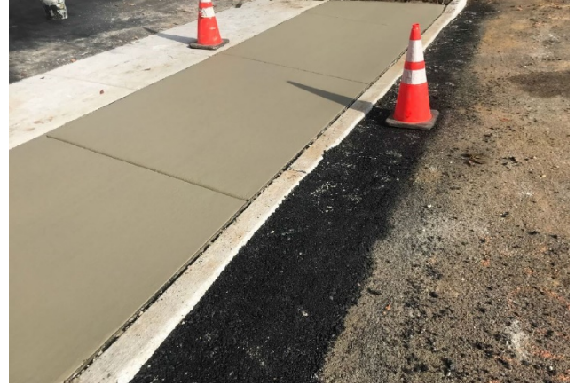
Figure 5: Concrete driveway placed
