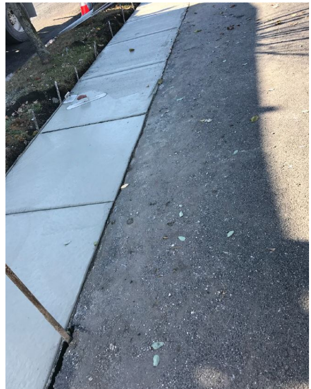
Figure 3: Concrete sidewalk
