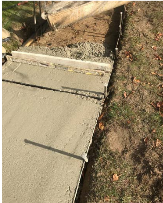
Figure 1: Concrete sidewalk placement
