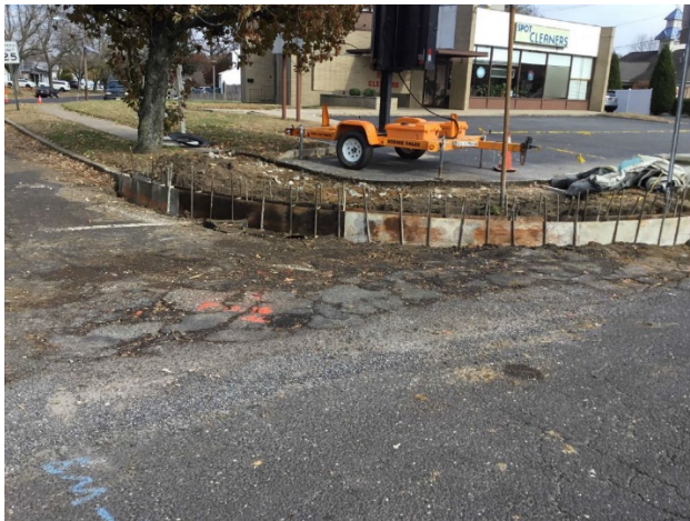
Figure 2: Concrete curb forms
