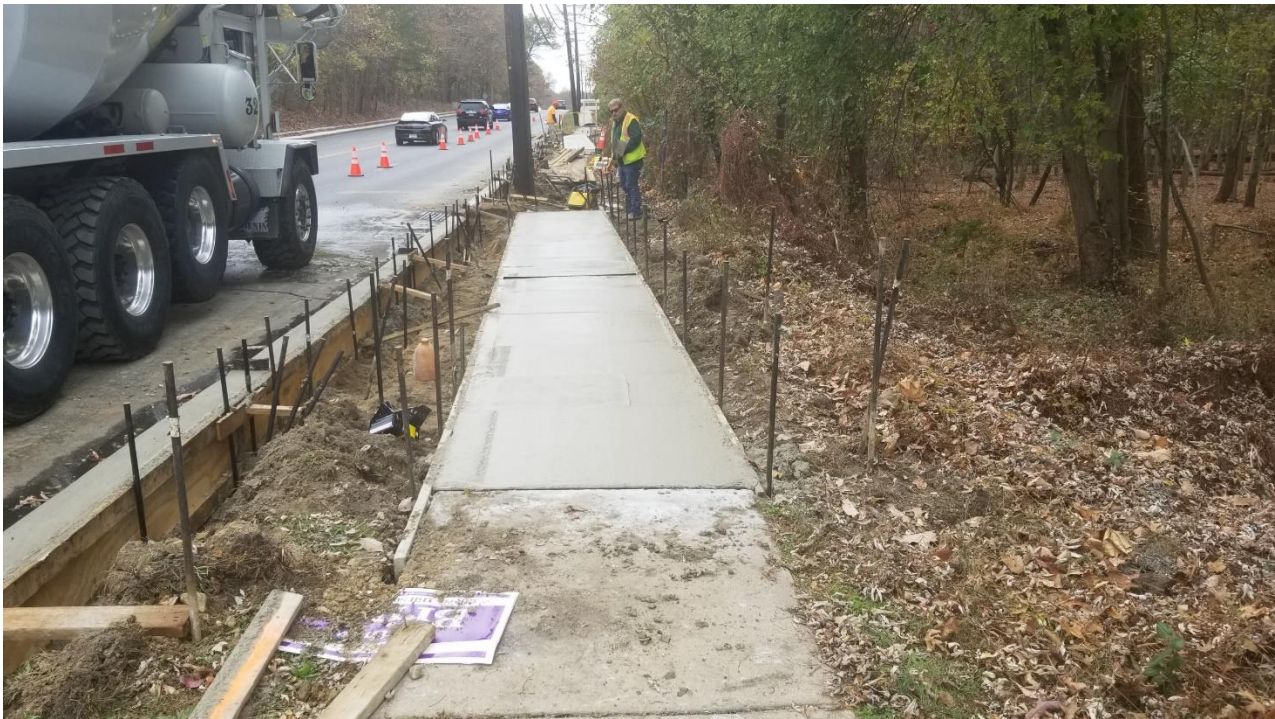
Figure 3. New sidewalk at Location 6 westbound. Note the utility pole will need to be relocated.
