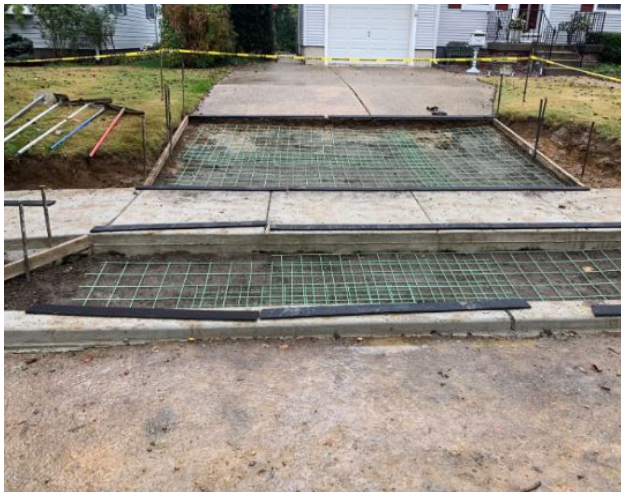
Figure 2: Reinforcement for concrete driveway
