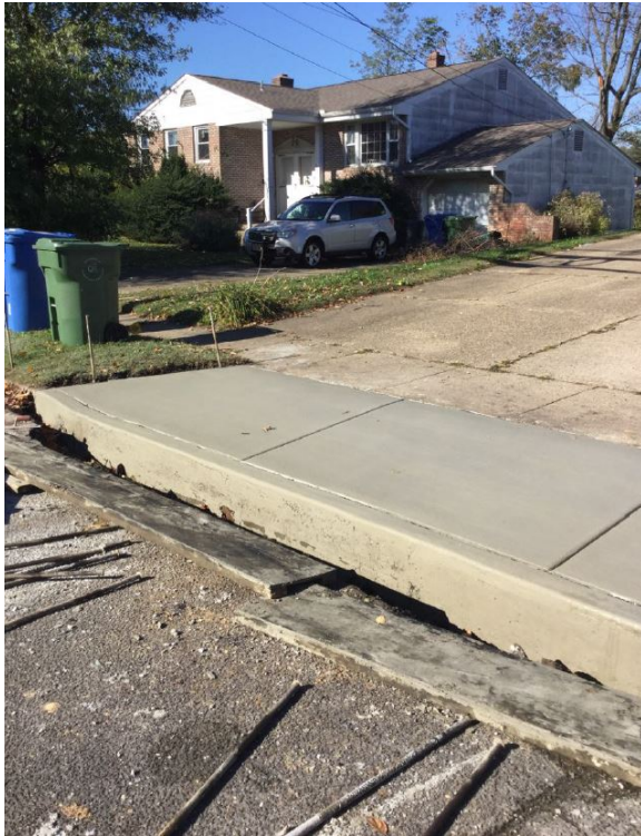
Figure 4: Concrete driveway placed
