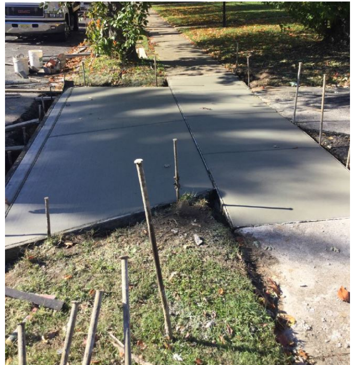
Figure 3: Concrete driveway and sidewalk palced
