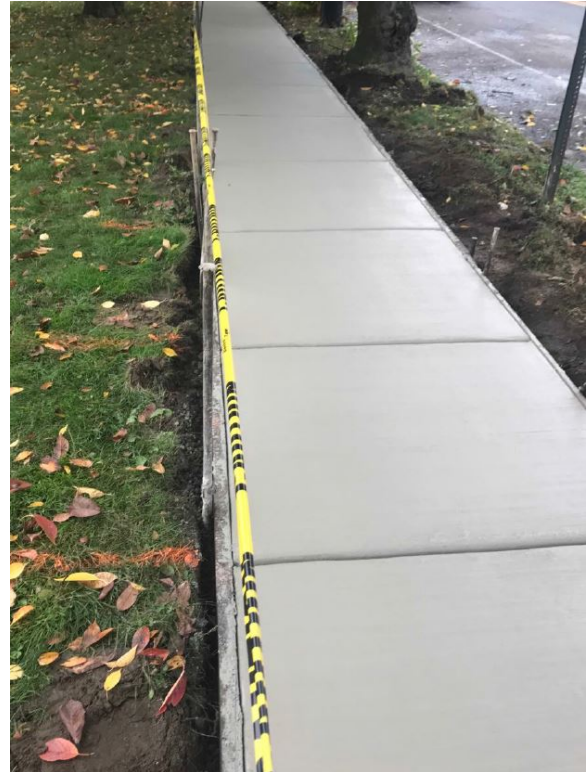
Figure 5: Concrete sidewalk placed
