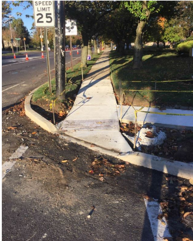
Figure 1: Concrete curb ramp
