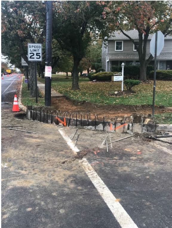
Figure 2: Concrete curb ramp area demolished
