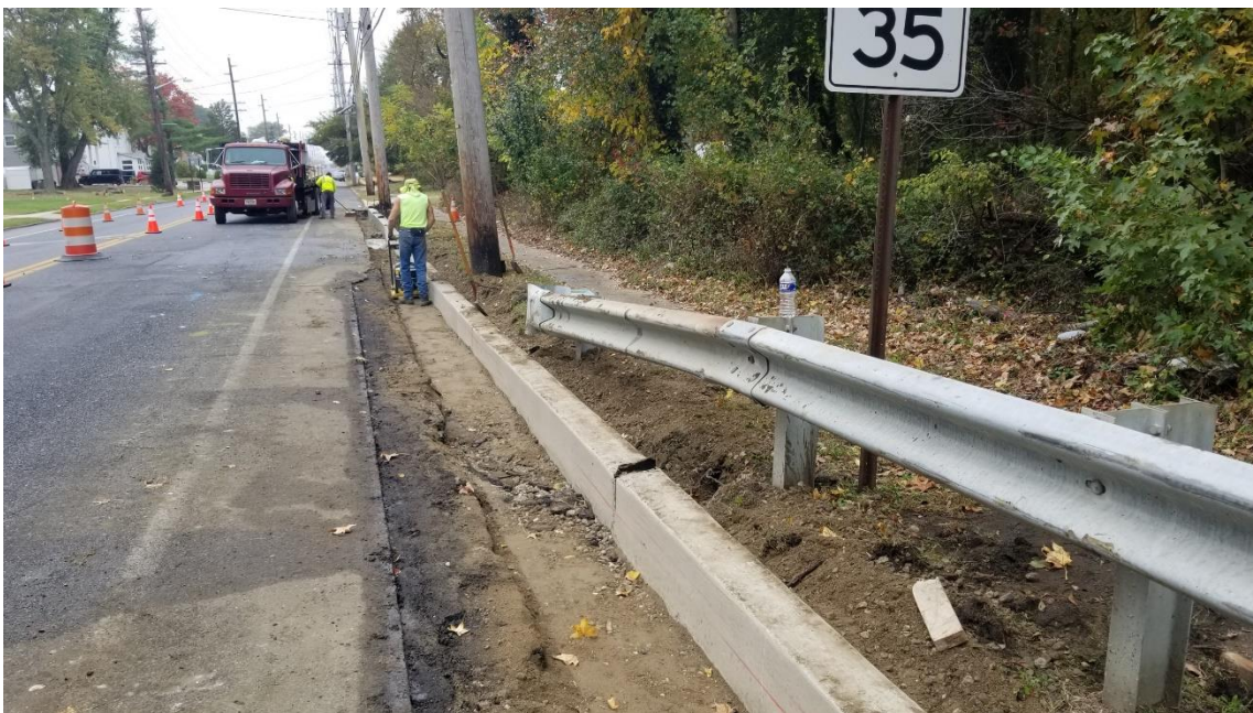
Figure 2. New curb at Location #3 westbound. Guiderail to be removed in this location.
