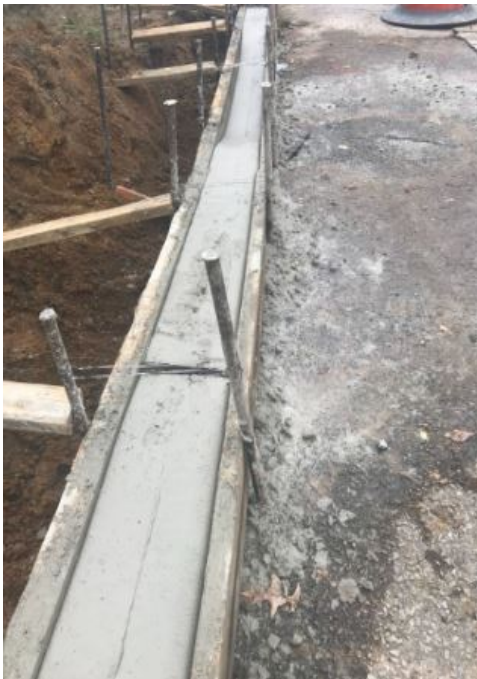
Figure 2: Concrete vertical curb placed
