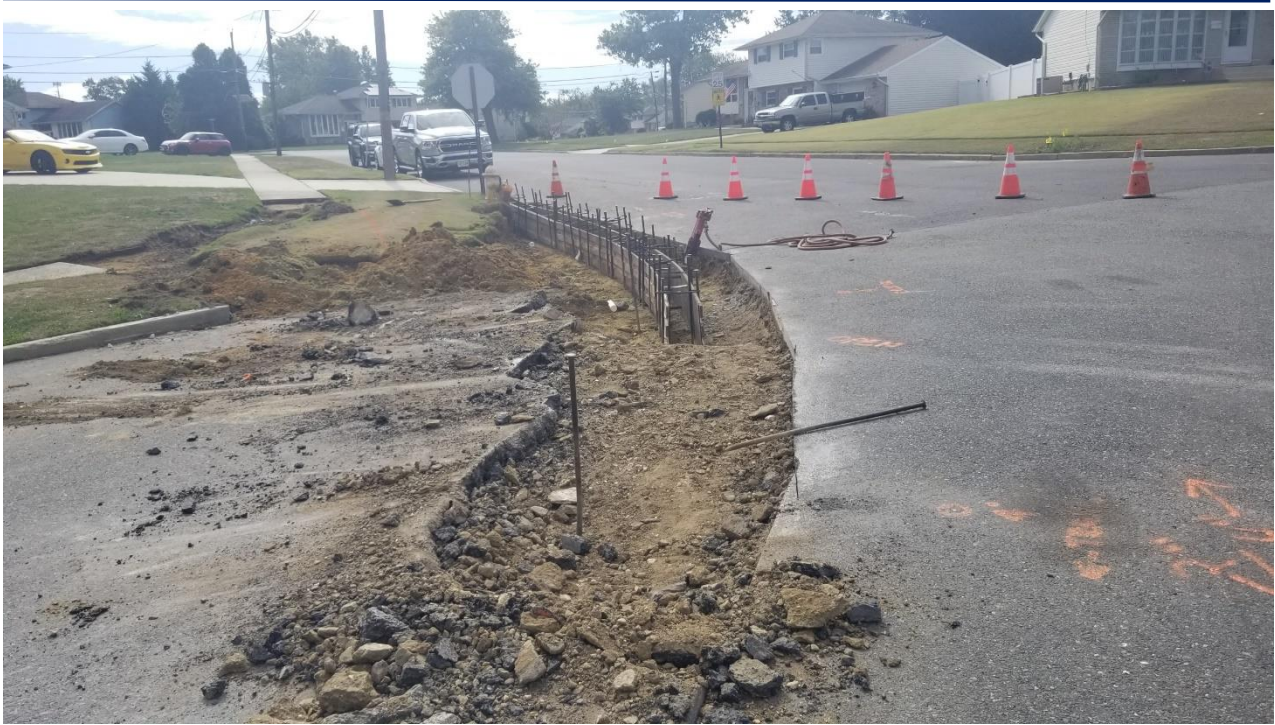
Figure 3. Lexa removed asphalt to extend the sidewalk and curb at the intersection of Albert Road and Evesham Road.
