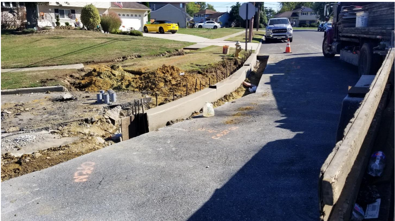
Figure 4. Lexa placed concrete curb at the intersection of Albert Road and Evesham Road.
