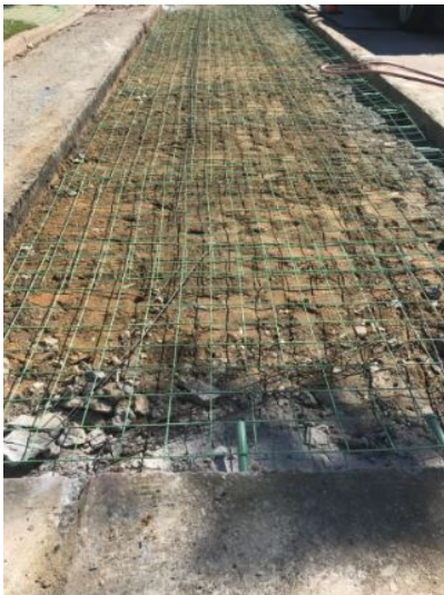
Figure 4: Reinforcement for concrete roadway repairs
