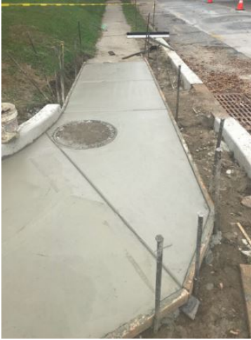
Figure 2: Concrete sidewalk placed
