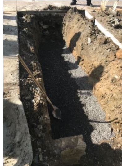
Figure 5: Trench for storm pipe installation
