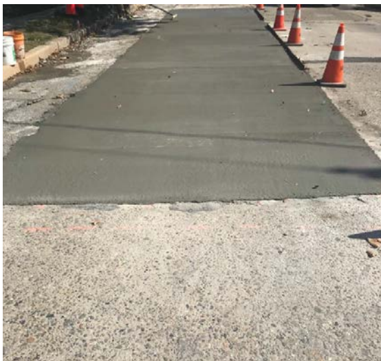
Figure 4: Concrete roadway repairs
