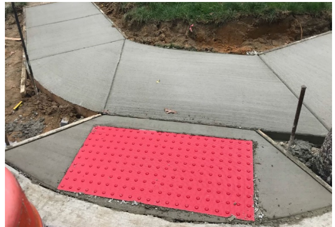
Figure 5: Concrete curb ramp placed
