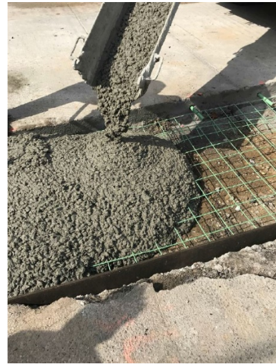
Figure 3: Concrete placement for road repair
