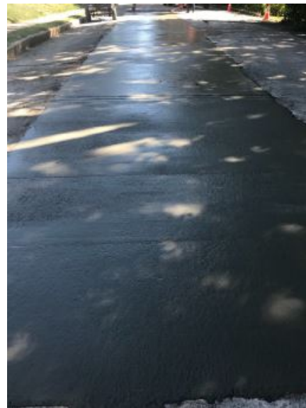
Figure 5: Concrete placed for roadway repairs
