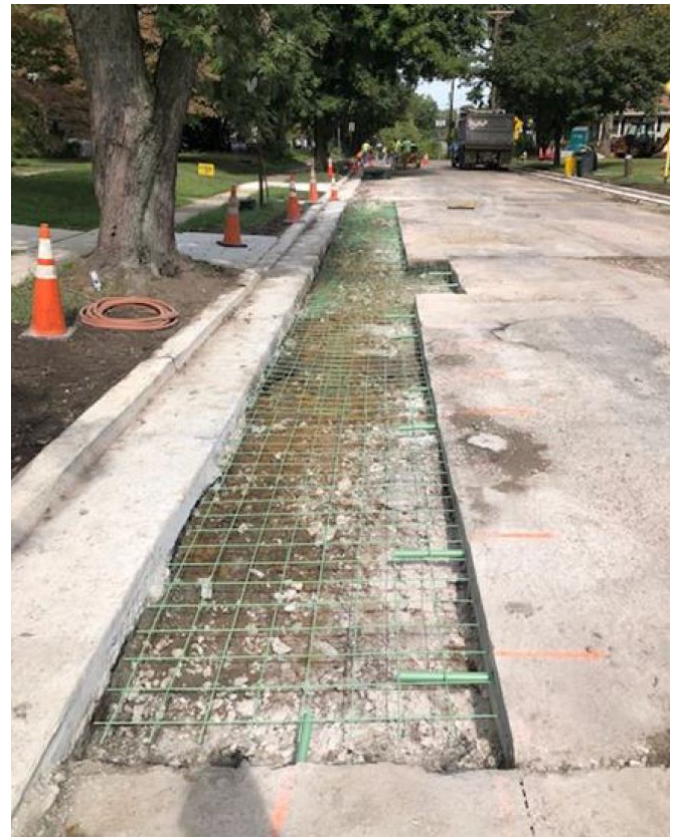
Figure 5: Concrete roadway repairs
