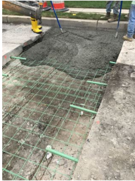
Figure 1: Concrete roadway repairs
