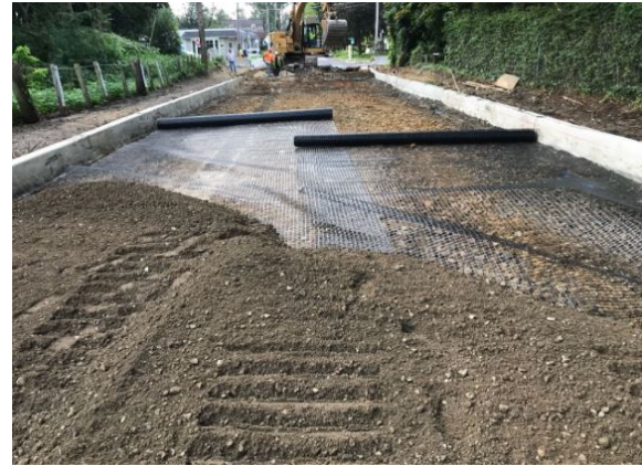
Figure 3: DGA and geogrid placement
