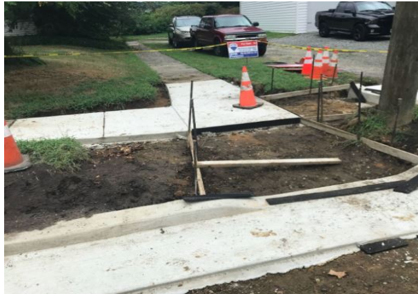
Figure 1: Concrete curb ramp reconstruction
