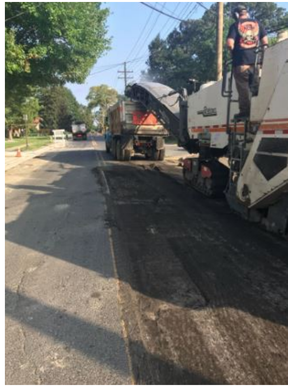
Figure 5: Milling operations along Hopkins Ave
