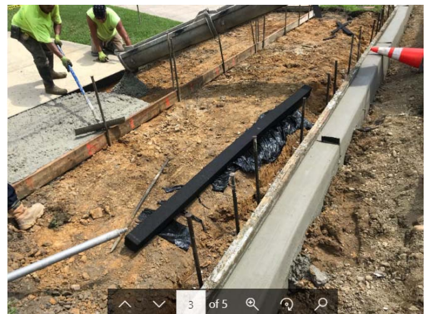
Figure 3: Concrete for 6" driveway being placed
