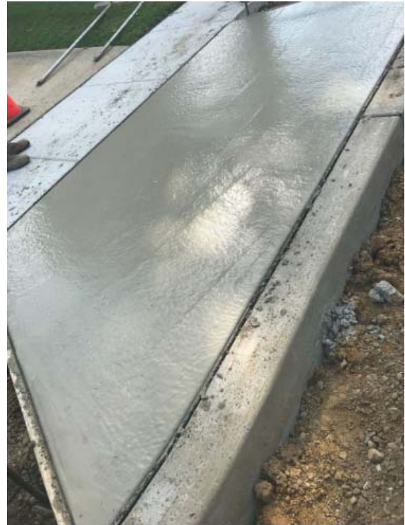
Figure 5: Concrete for 6" driveway being placed
