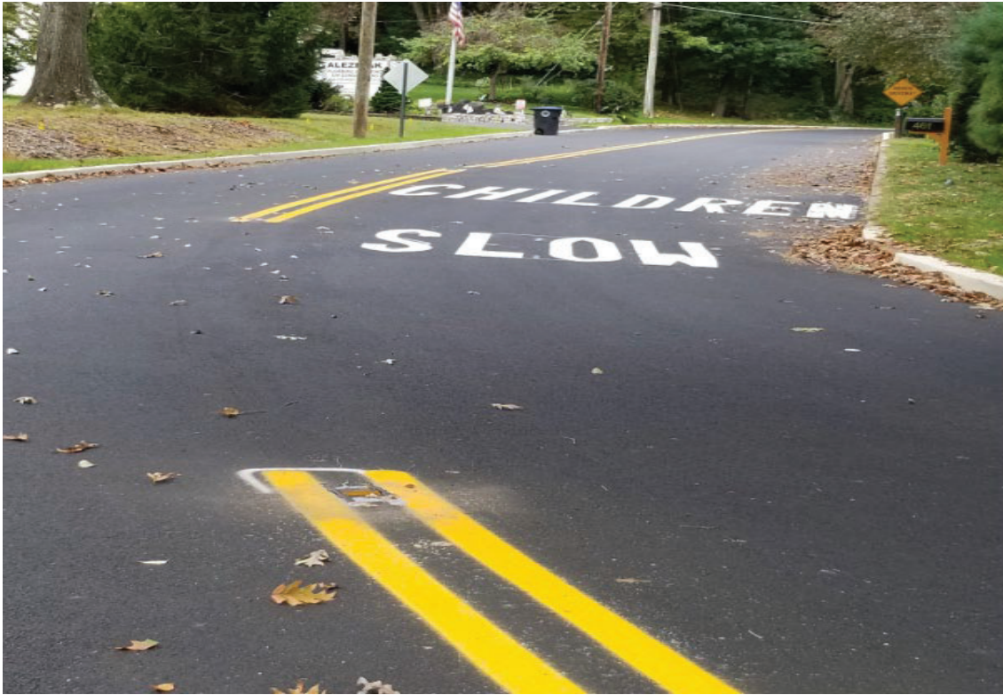
Figure: 2 –Repaint Centerlines and Traffic control and Signage installed for entire road (If and where directed)
