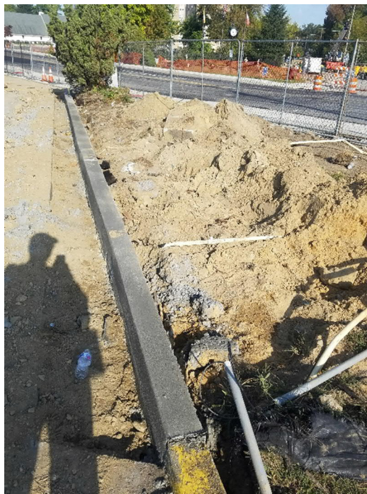
Vertical curb poured at bank parking lot
