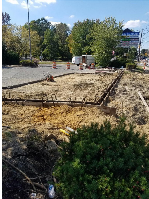
Vertical curb forms re-establishing the parking lot
