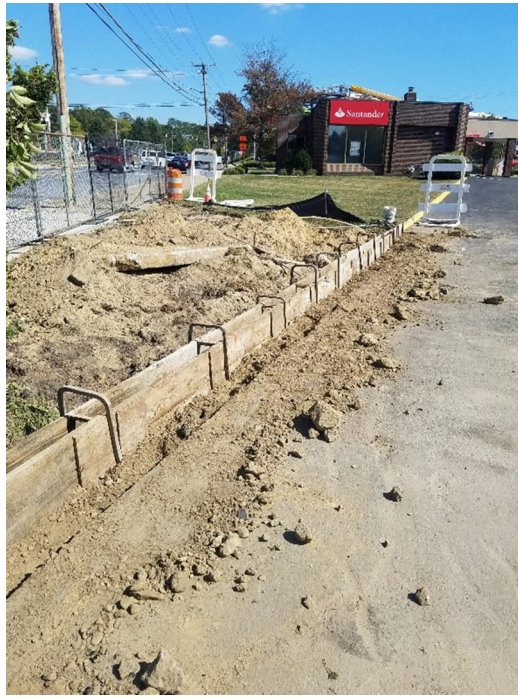
Vertical curb formed at the bank parking lot and temporary walkway removed
