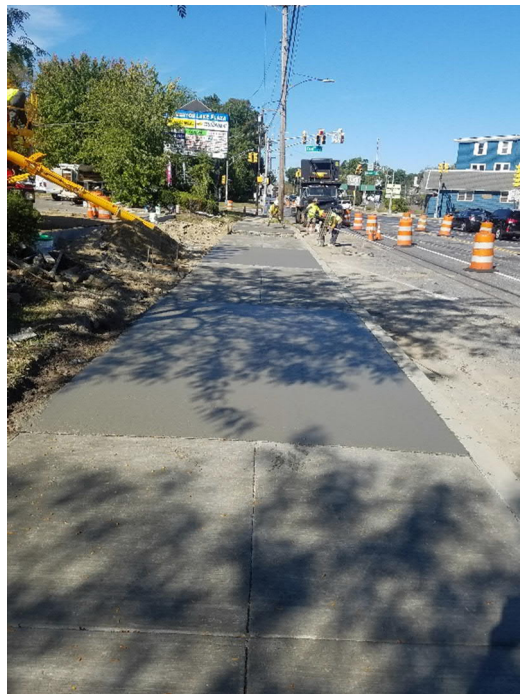
Sidewalk poured and tied into existing sidewalk
