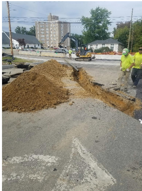
Removing temporary water line
