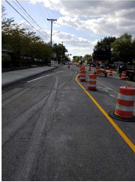
Old stripes and markings removed, new traffic pattern for stage 4B installed
