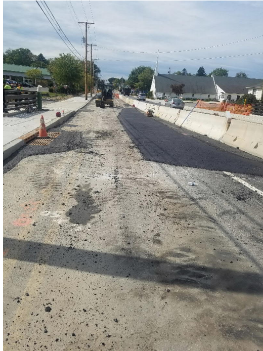
Leveling course of asphalt installed where needed
