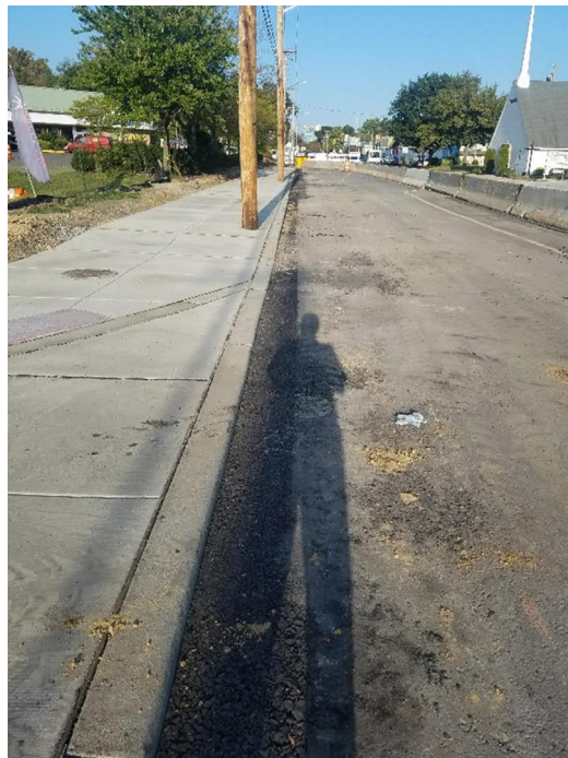
Vertical curb and sidewalk
