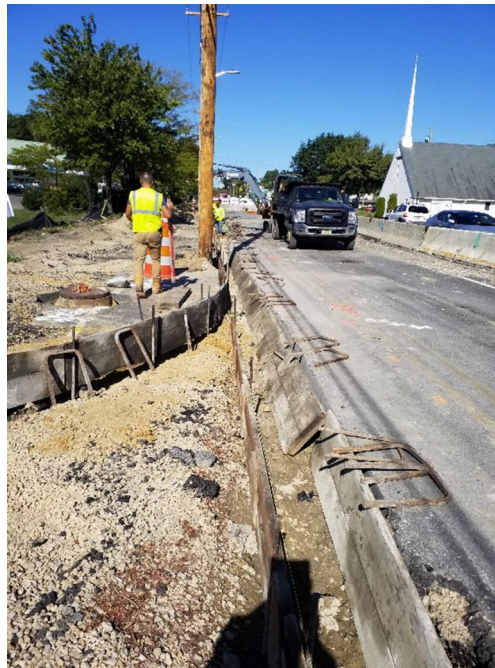
Forming for concrete curb & sidewalk
