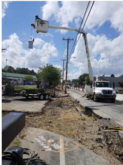
Power Lines restored to original location
