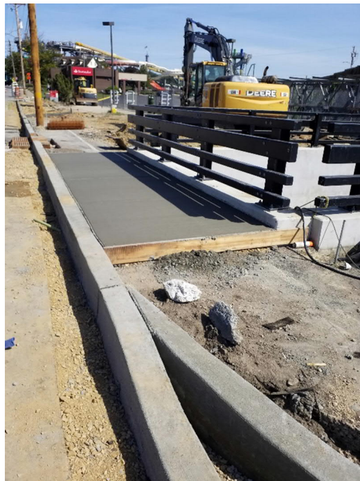
Vertical curb and sidewalk
