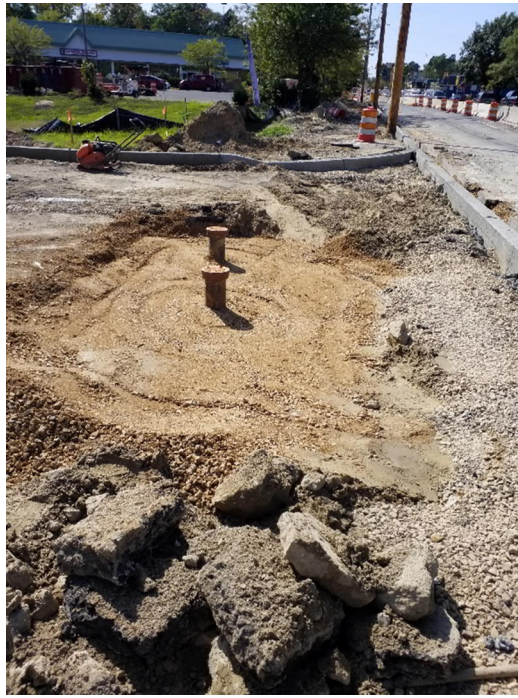
Valve boxes raised to grade
