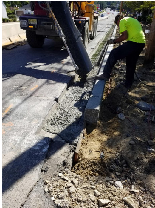
Concrete roadway repair
