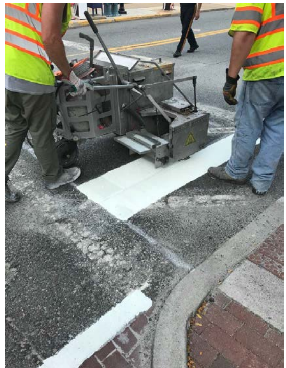
Figure 3: Installation of new striping
