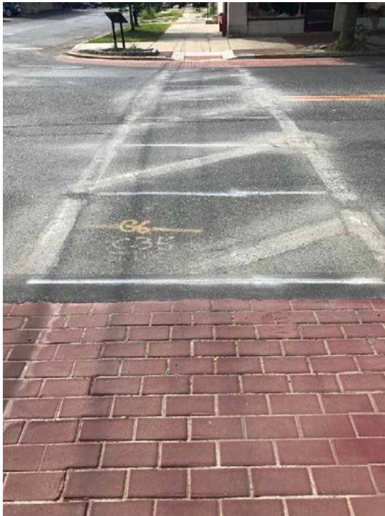
Figure 2: Existing striping removed
