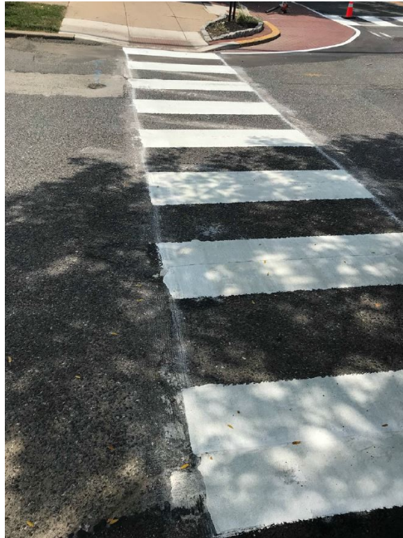
Figure 1: New striping installed
