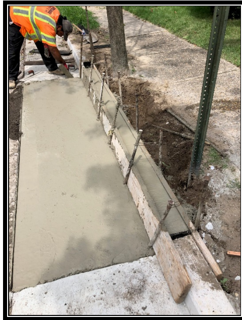
Figure 2: All damaged gutter replaced by contractor.
