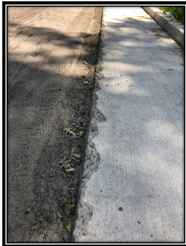
Figure 1: New gutter damaged by milling machine.
