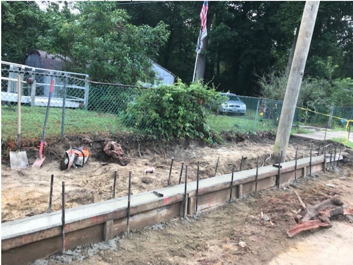
Figure: 2 – Reconstruct Curb and Handicap Ramp starting near Cottage Ave and Scott ave (If and where directed)
