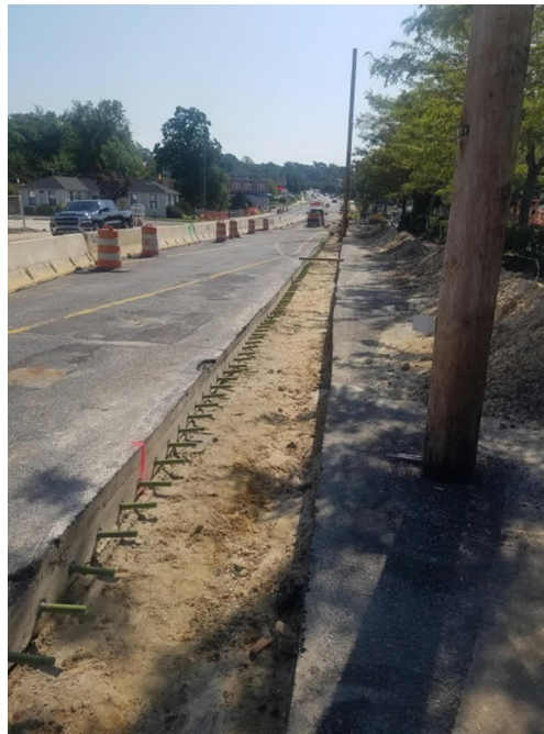
1 ½" x 18" steel bars epoxied in place
