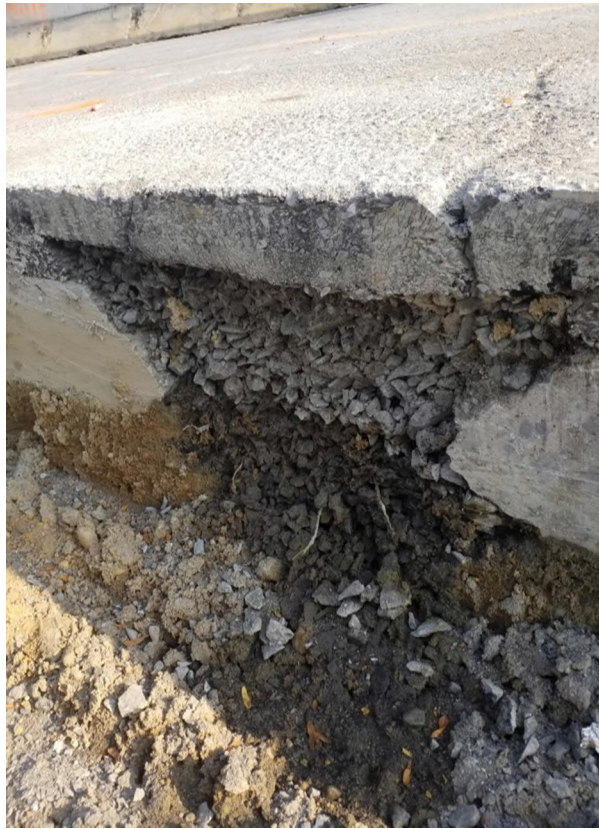
Concerns about existing transverse patch repairs
