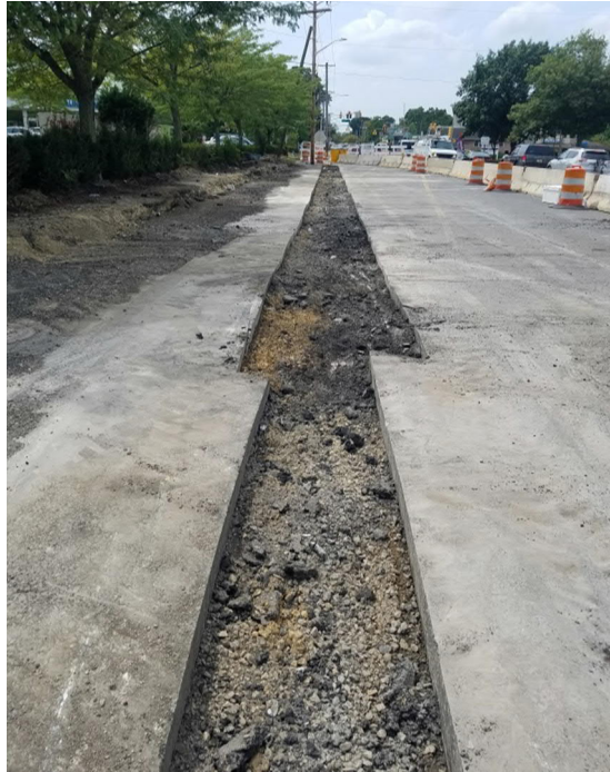
Asphalt and concrete removed
