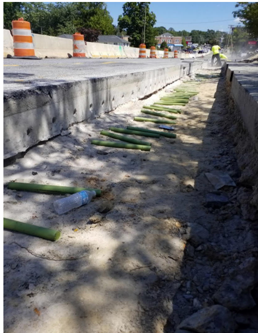
Drilled holes for dowels
