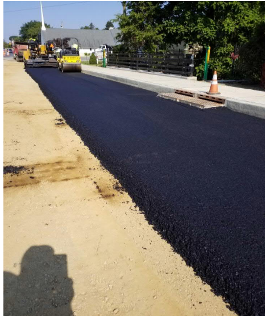
Paving first of two lifts of base
