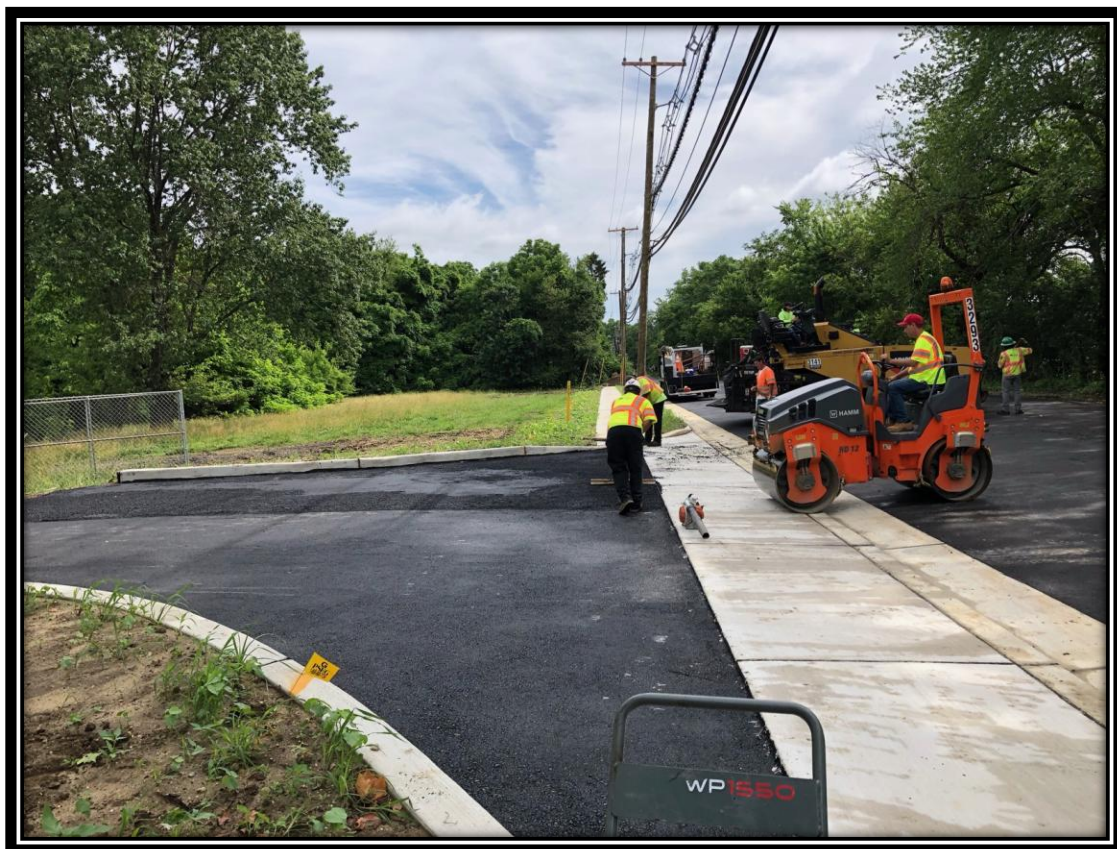
Figure: 1 – Installation of HMA driveway along the westbound lane at the eastern entrance to the proposed First Montgomery Development
