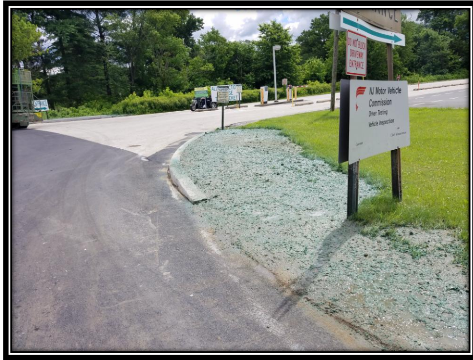
Figure: 2 – Installation of topsoil and hydro seed along the eastbound lane at the main entrance to the department of motor vehicles
