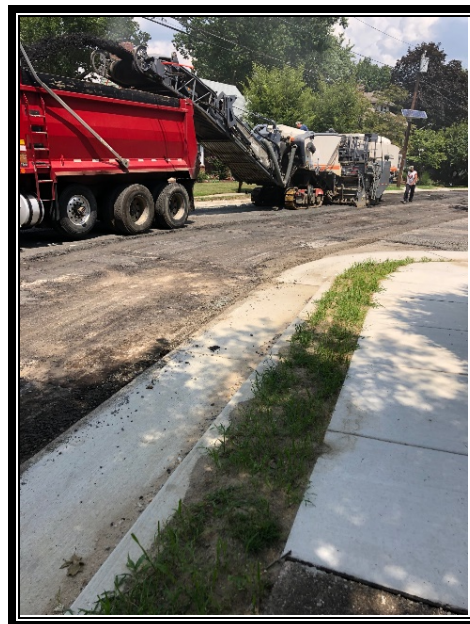
Figure 3: Milling existing asphalt from concrete base course.
