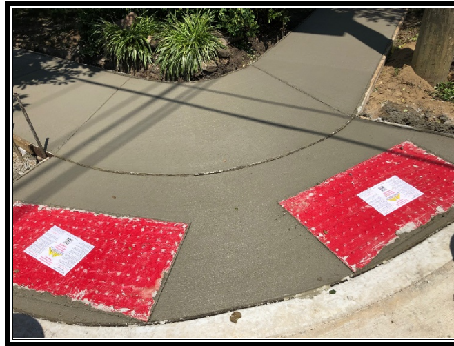
Figure 2: New handicap ramps at the intersection of Crystal Lake and Avondale Avenues.
