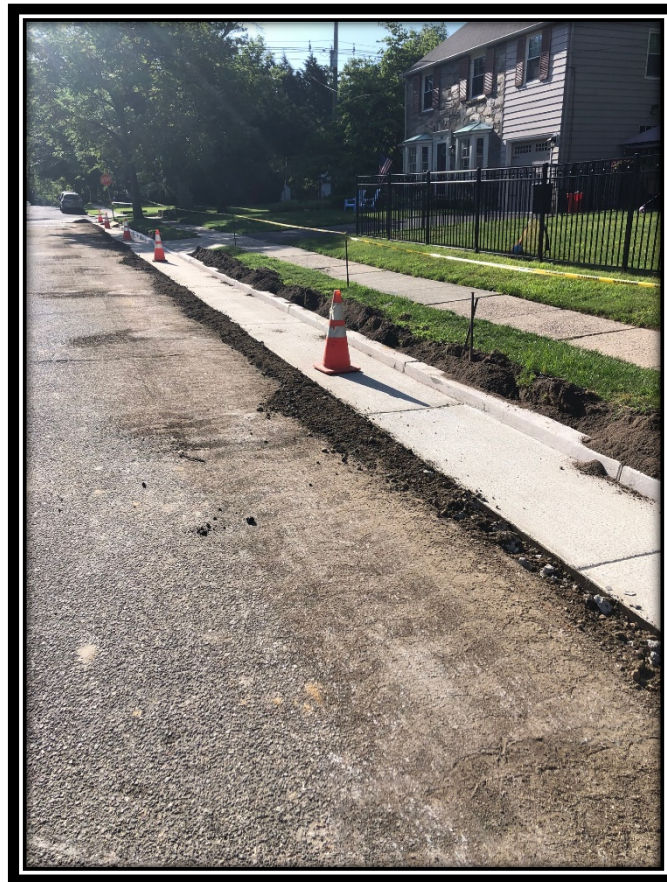
Figure 1: Completed curb and gutter on Avondale Avenue.
