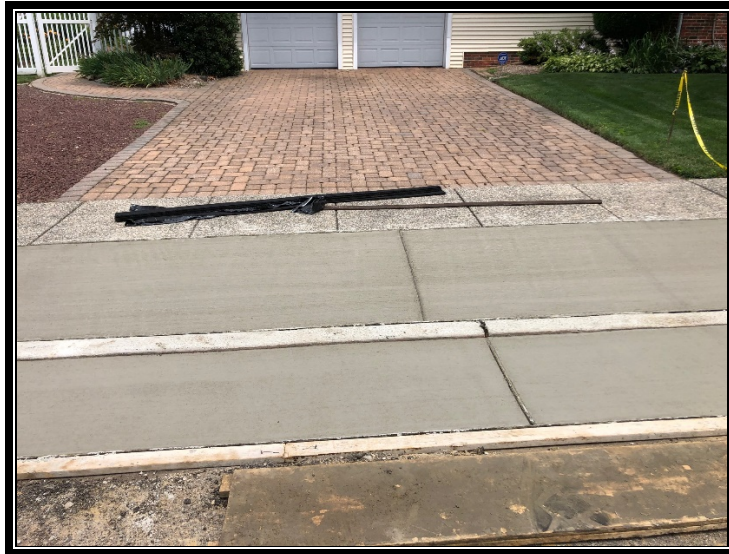
Figure 2: New concrete driveway apron and gutter.
