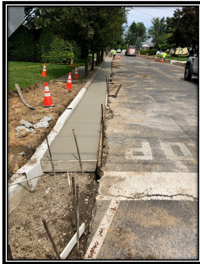
Figure 1: New curb and gutter on Breslin Avenue.
