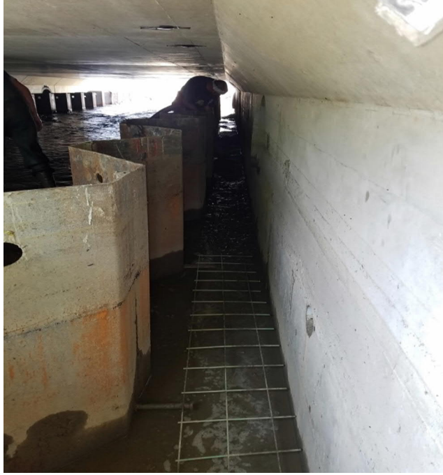
Poured concrete "cap" between culvert walls and permanent sheeting
