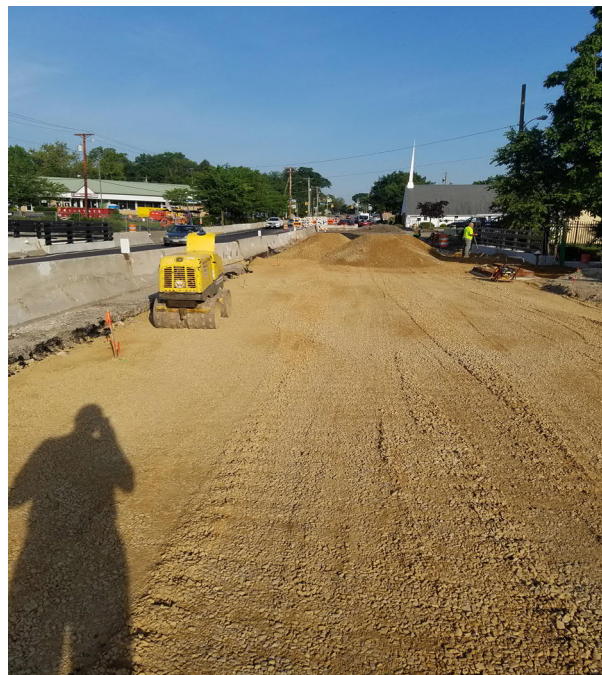
DGA placed and compacted
