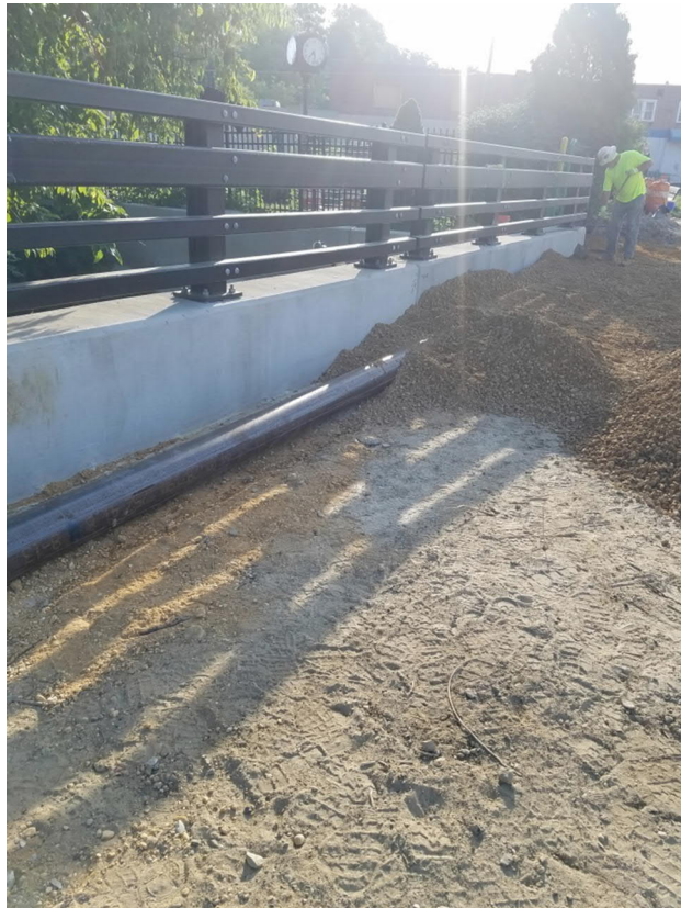
Steel casing covered with DGA
