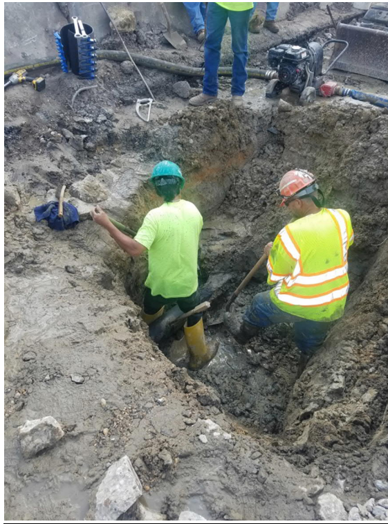
Water main break repair
