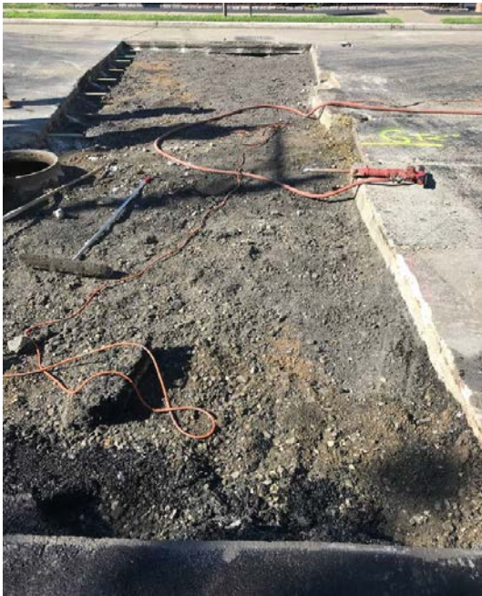
Figure 2: Proposed concrete road reconstruction area excavated
