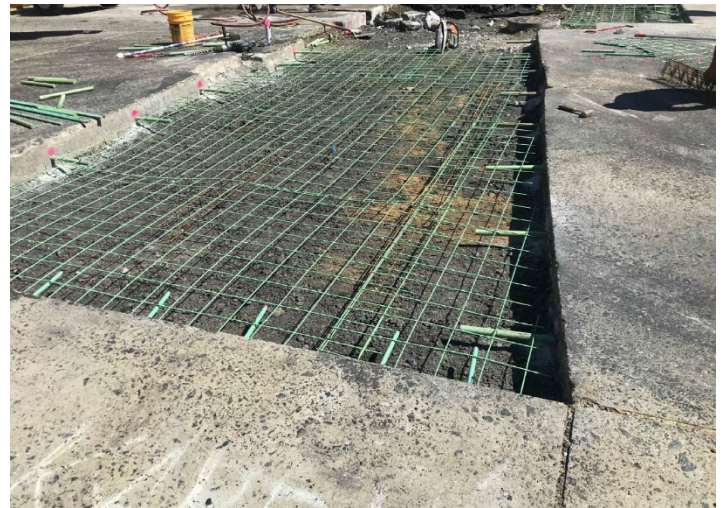
Figure 3: Reinforcement set for concrete road reconstruction area
