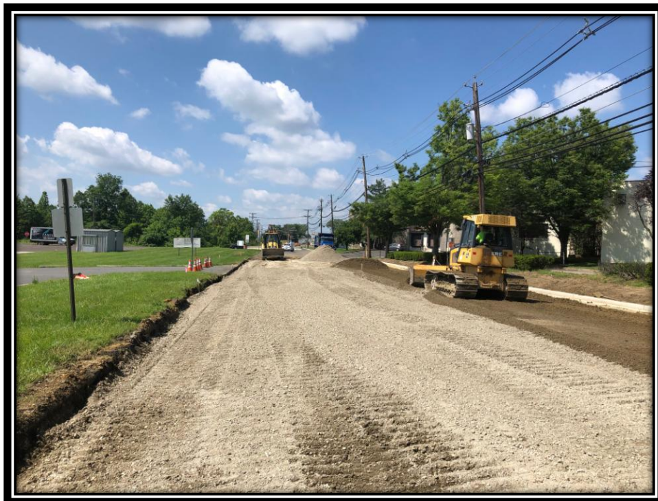
Figure: 3 – Installation of 6" thick dense graded aggregate base course along the frontage of the Department of Motor Vehicles
