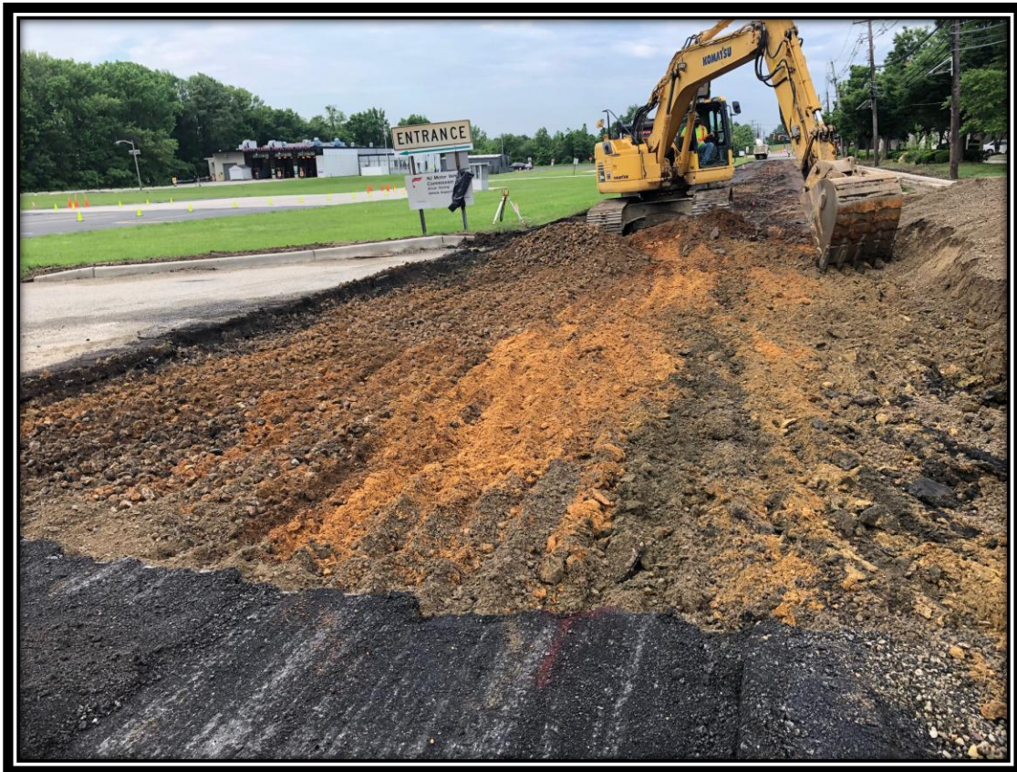
Figure: 1 – Roadway excavation along the frontage of the Department of Motor Vehicles
