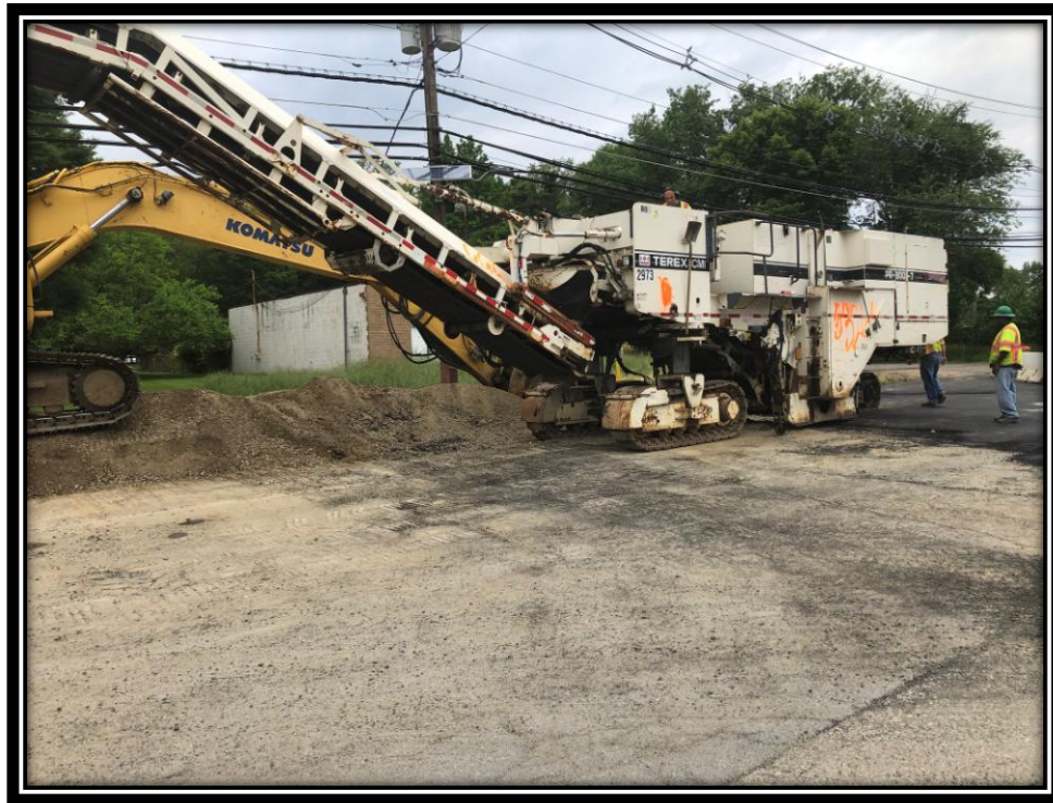
Figure: 2 – Milling of existing asphalt along the westbound lane along the frontage of the Department of Motor Vehicles
