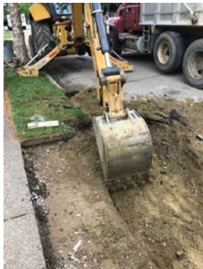
Figure 2: Demolition of Concrete Curb
