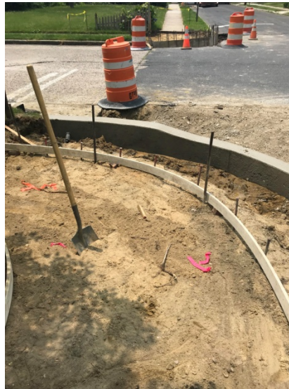
Figure 1: Concrete Vertical Curb Placed; 4" Sidewalk Formed Up
