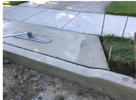
Figure 3: Concrete Driveway, Reinforced, 6" Thick
