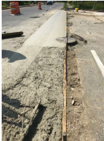
Figure 1: Concrete placement for swale at Cuthbert Boulevard
