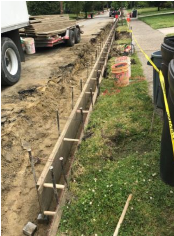
Figure 2: Concrete curb formed up
