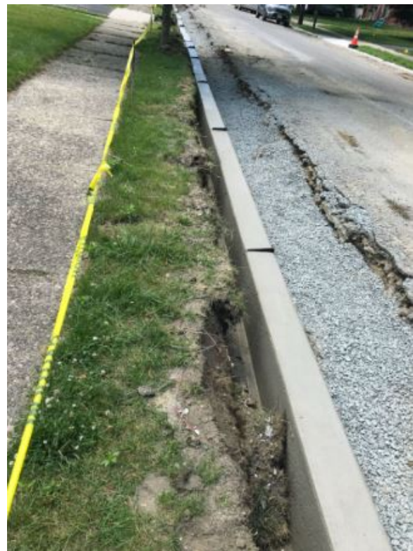
Figure 3: Concrete vertical curb, expansion joints included
