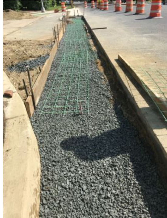
Figure 5: Reinforcement for concrete swale at Cuthbert Boulevard
