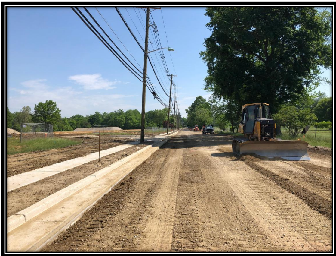
Figure: 1 – Fine grading of previously installed dense graded aggregate in preparation for base paving
