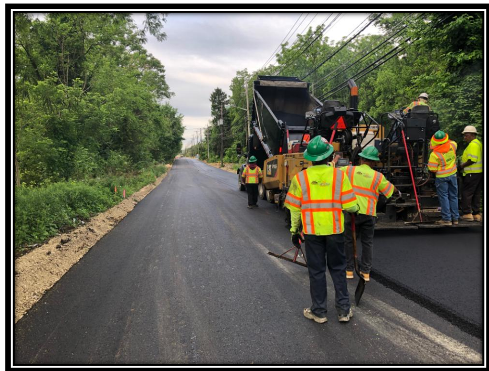
Figure: 3 – Installation of HMA 12.5M64 intermediate course along the westbound lane between Chapel Avenue and the Department of Motor Vehicles entrance
