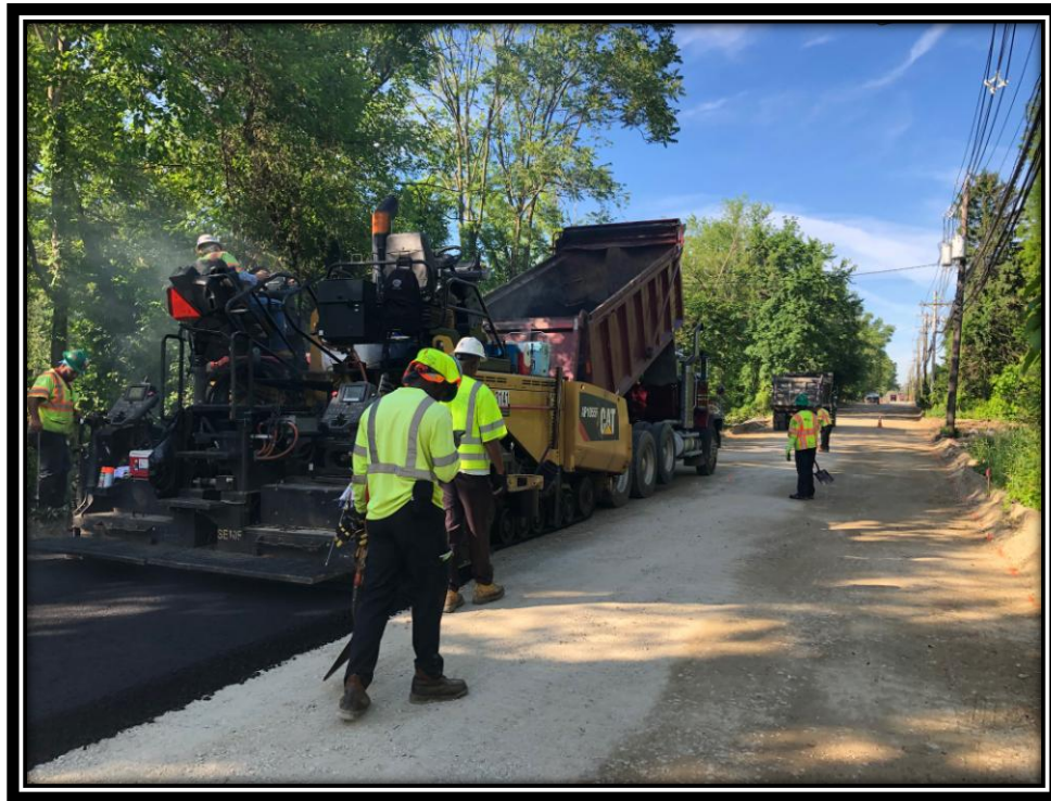
Figure: 2 – Installation of HMA 25M64 base course along the eastbound lane between Chapel Avenue and the Department of Motor Vehicles entrance
