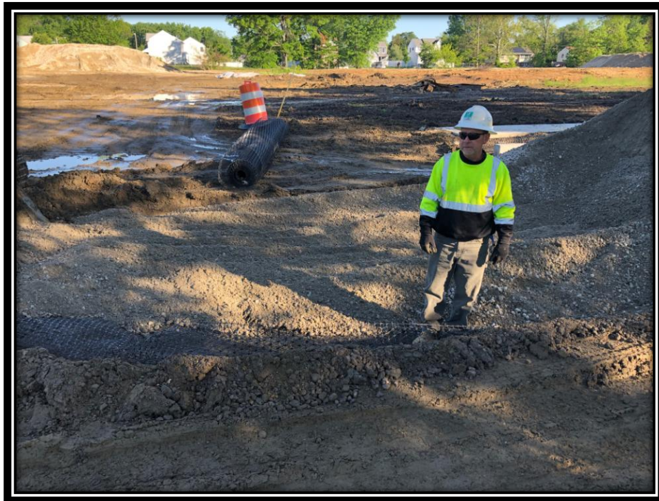
Figure: 3 – Installation of dense graded aggregate and geogrid prior to fine grading
