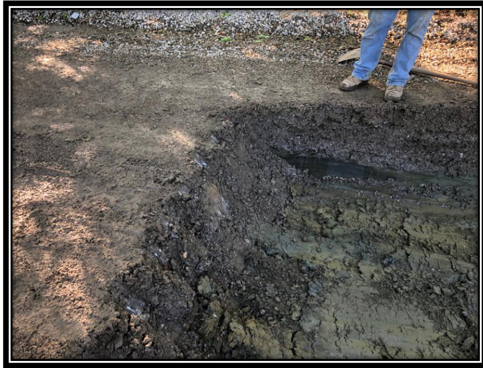
Figure: 2 – Over excavation of unsuitable subbase prior to installation of additional dense graded aggregate
