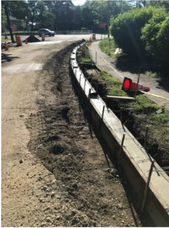
Figure 2: Concrete vertical curb poured
