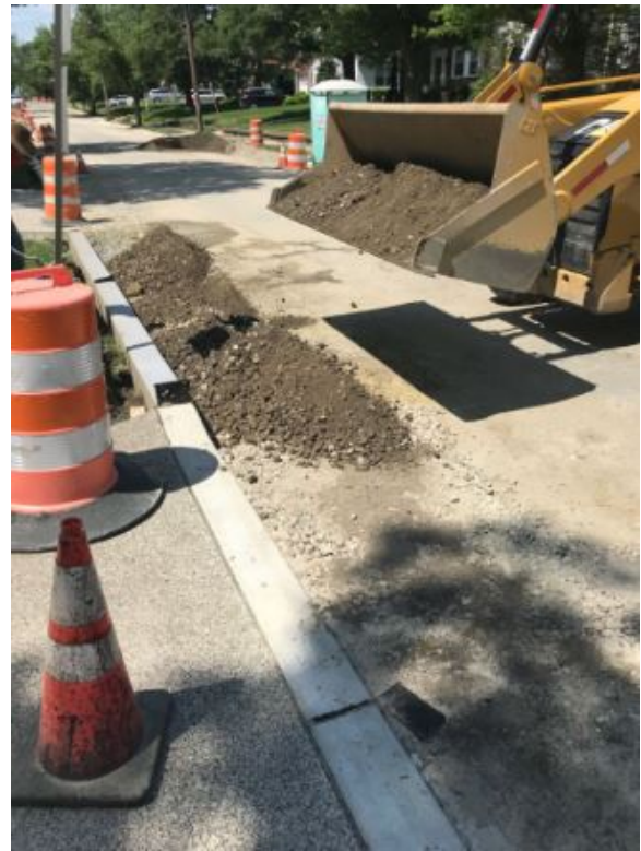
Figure 3: Concrete installed, temporary roadway restoration
