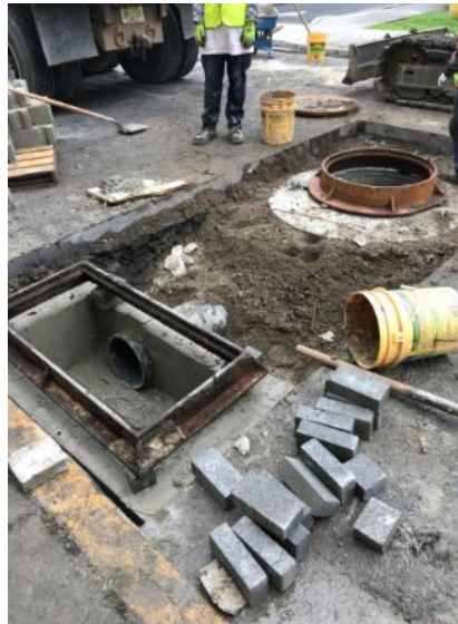
Figure 1: Storm sewer installation
