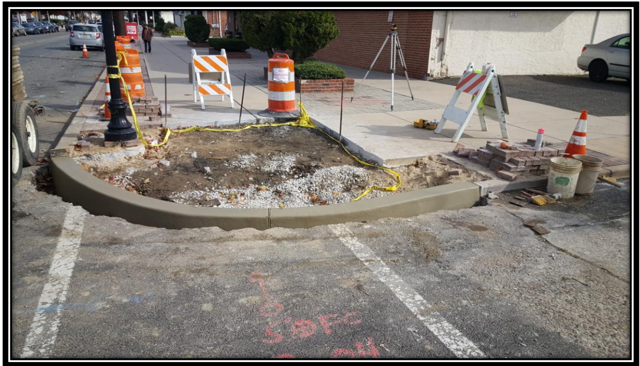
Figure: 2 – Installation of concrete curb at the southeast corner of the intersection with 49 th Street along the eastbound lane
