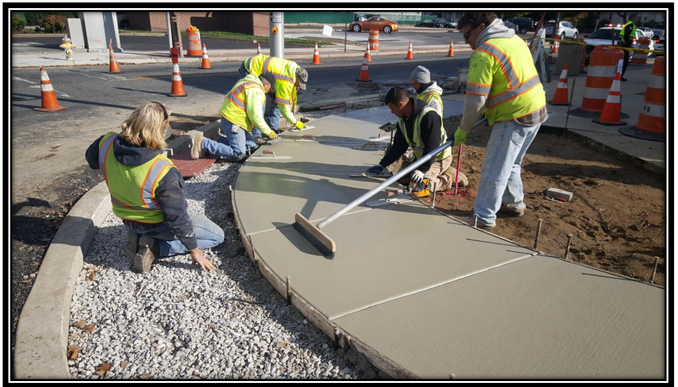
Figure: 1 – Installation of a concrete sidewalk at the southwest corner of the intersection with Browning Road along the eastbound lane
