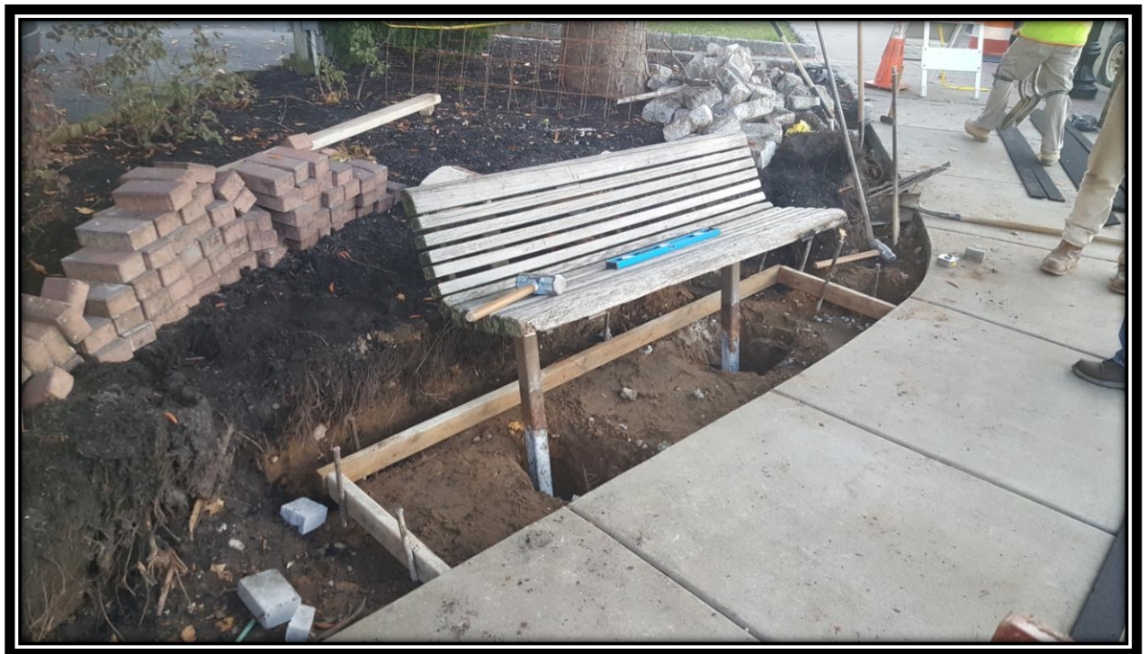
Figure: 3 – Resetting of an existing bench at the northeast corner of the intersection with Browning Road along the westbound lane
