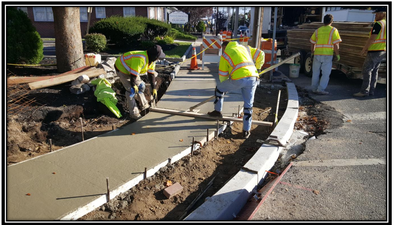
Figure: 1 – Installation of a concrete sidewalk at the northeast corner of the intersection with Browning Road along the westbound lane
