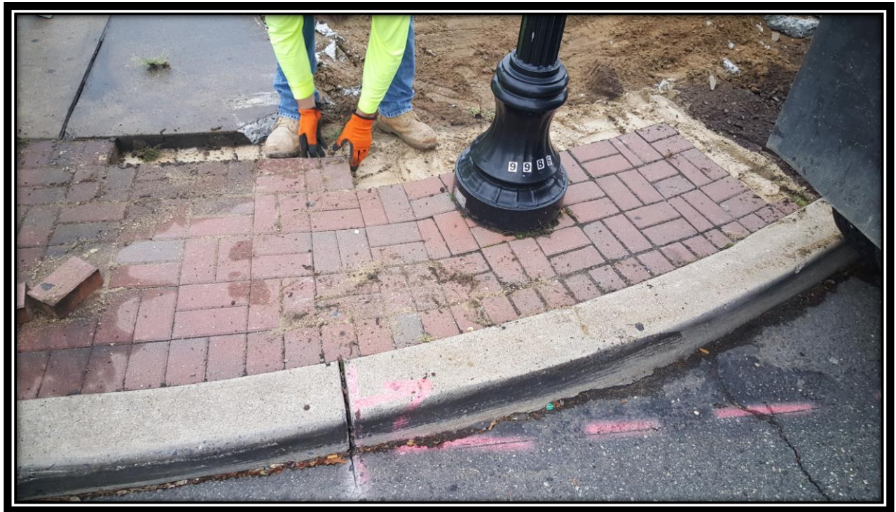
Figure: 2 – Resetting of brick pavers at northwest corner of the intersection with 46th Street along the westbound lane
