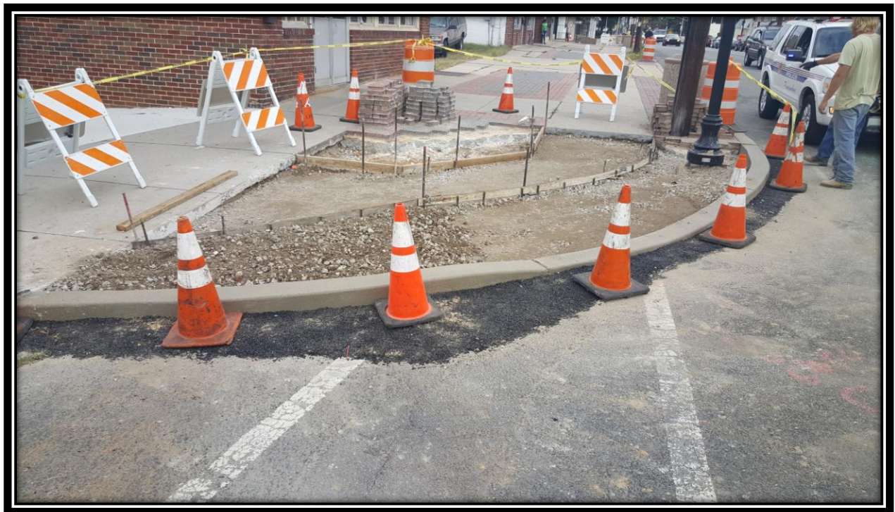
Figure: 3 – Installation of concrete curb at the northeast corner of the intersection with 48 th Street along the westbound lane
