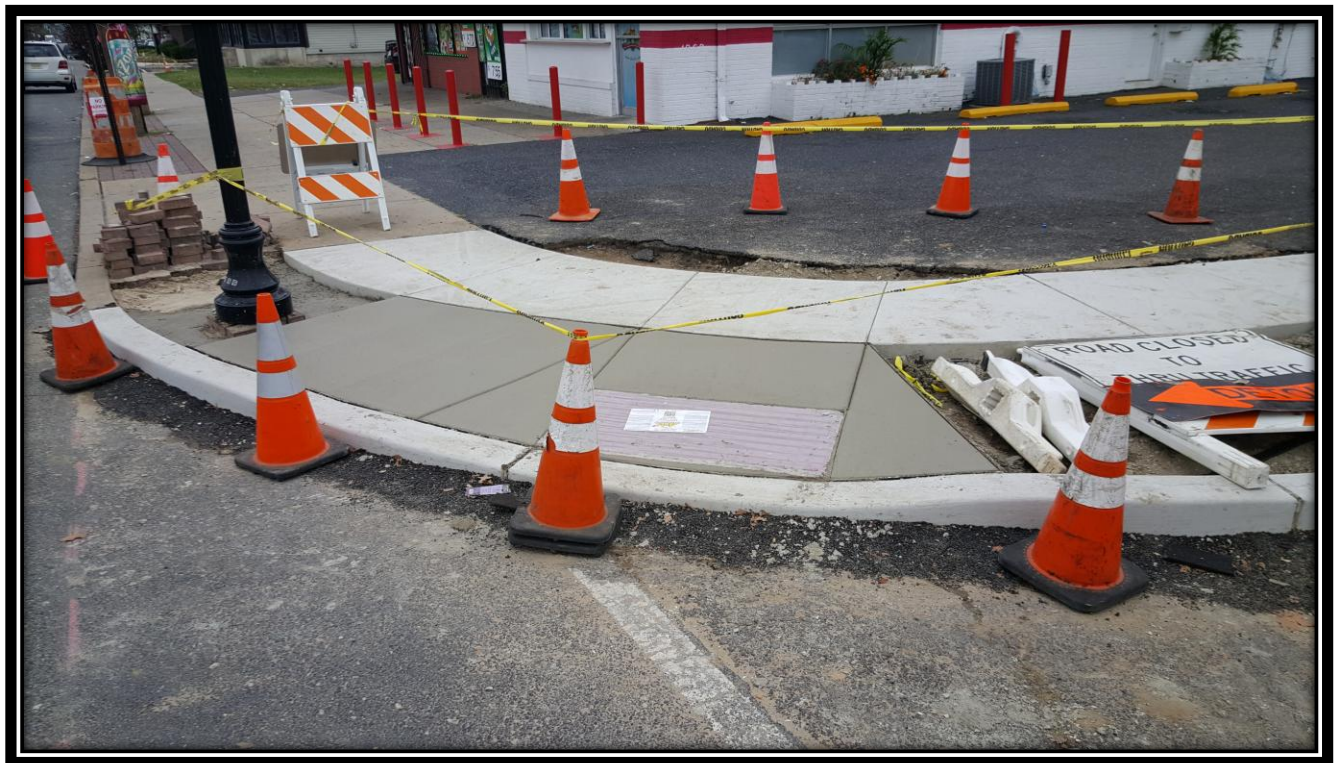
Figure: 1 – Installation of a concrete ADA ramp at the northwest corner of the intersection with 48 th Street along the westbound lane
