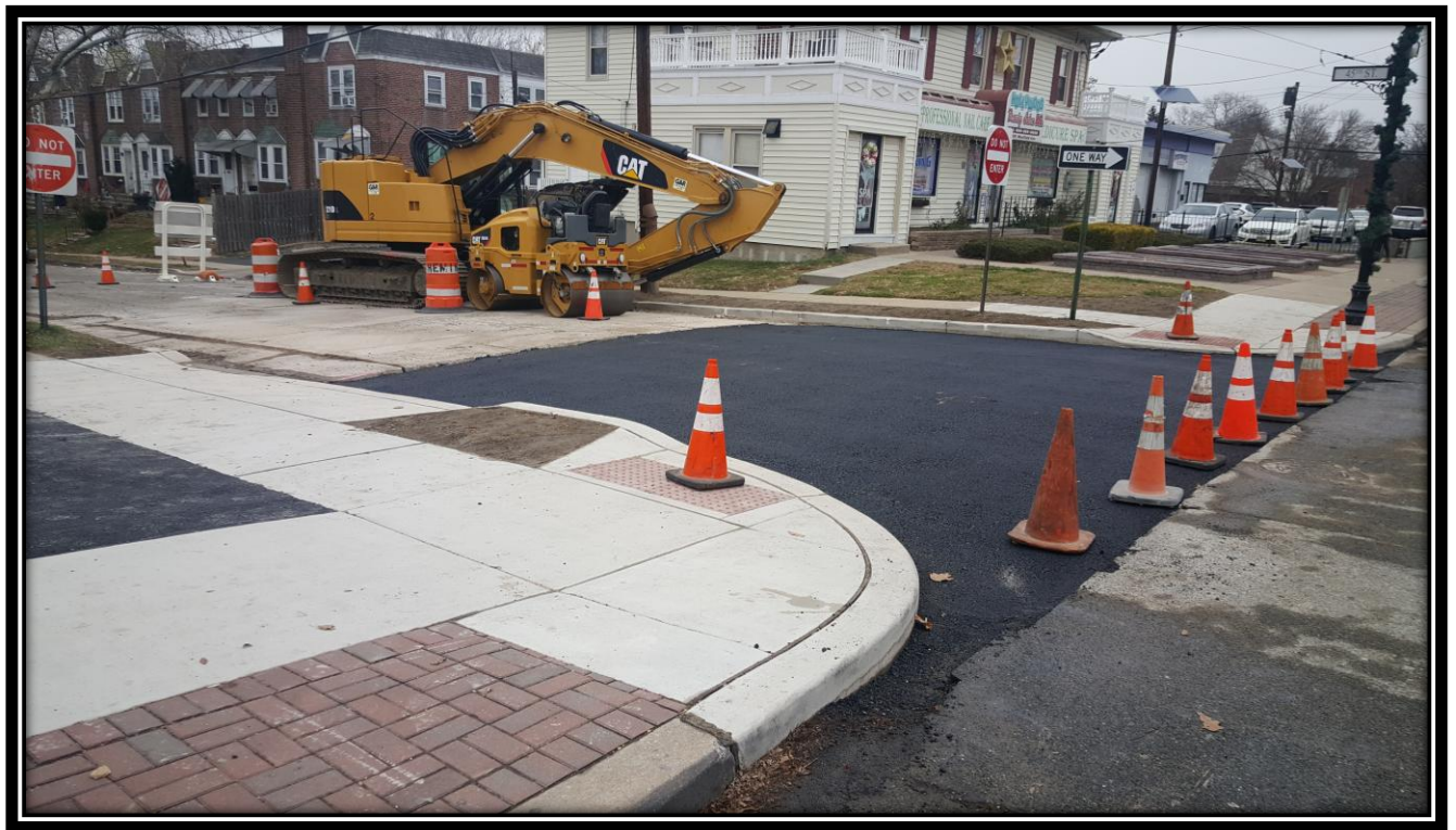
Figure: 1 – Installation of HMA 19M64 base course at the intersection with 45 th Street along the westbound lane
