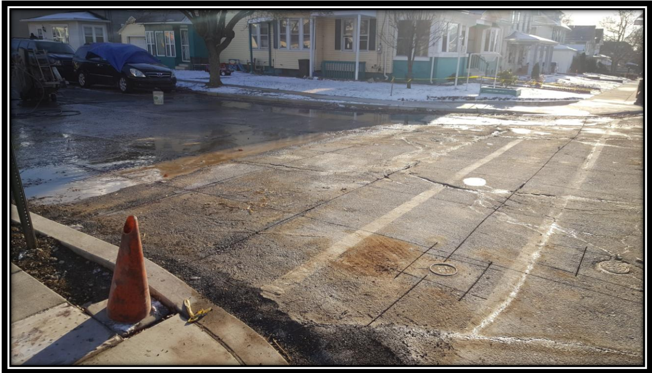
Figure: 2 – Saw cutting of the existing roadway at the intersection with 44 th Street along the eastbound lane
