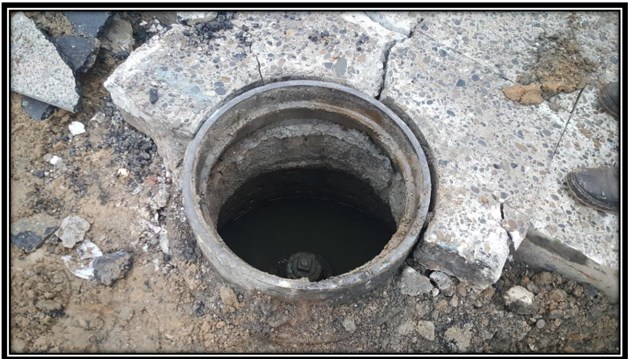
Figure: 3 – Resetting of the existing water manhole in the intersection with 47 th Street along the eastbound lane
