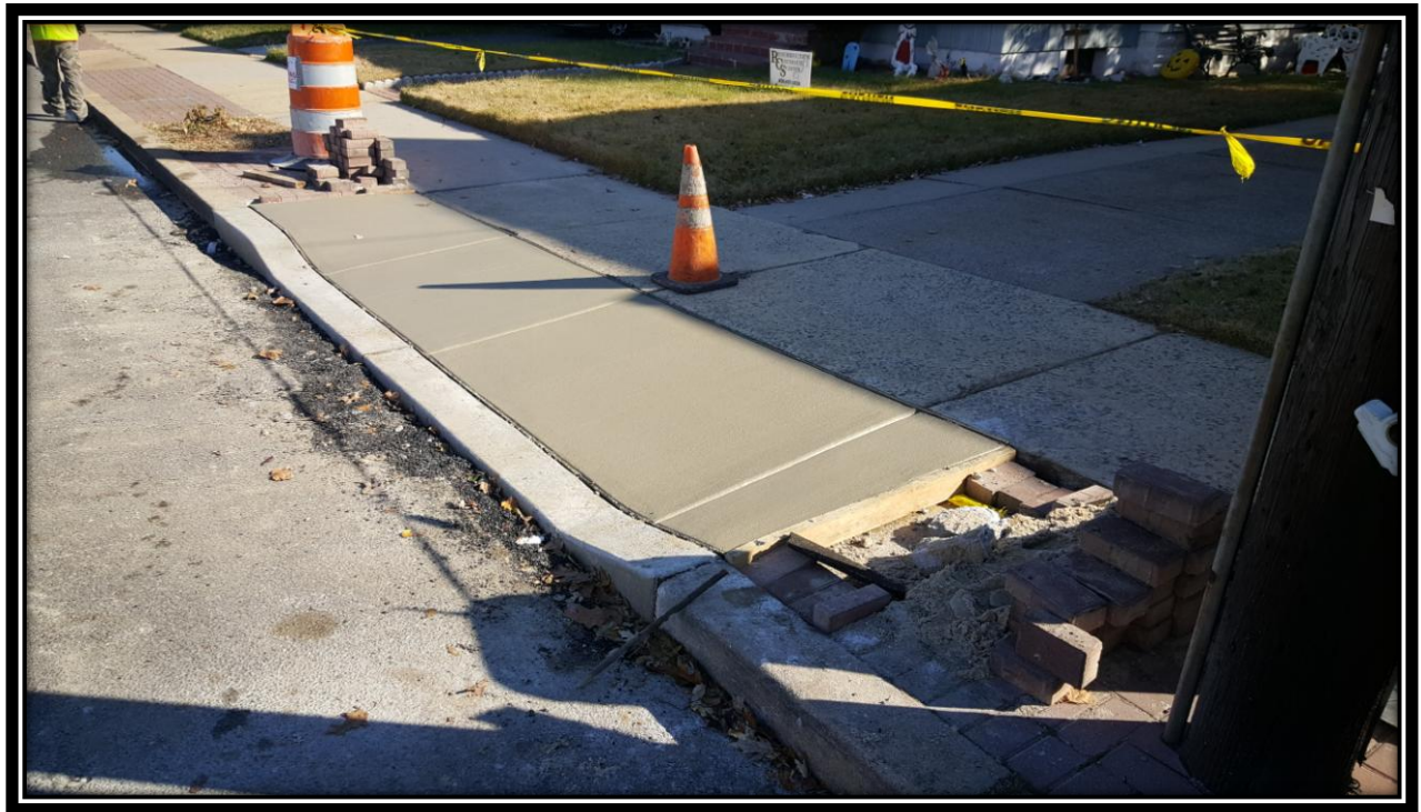
Figure: 2 – Installation of concrete driveway apron between 45 th Street and 46 th Street along the eastbound lane
