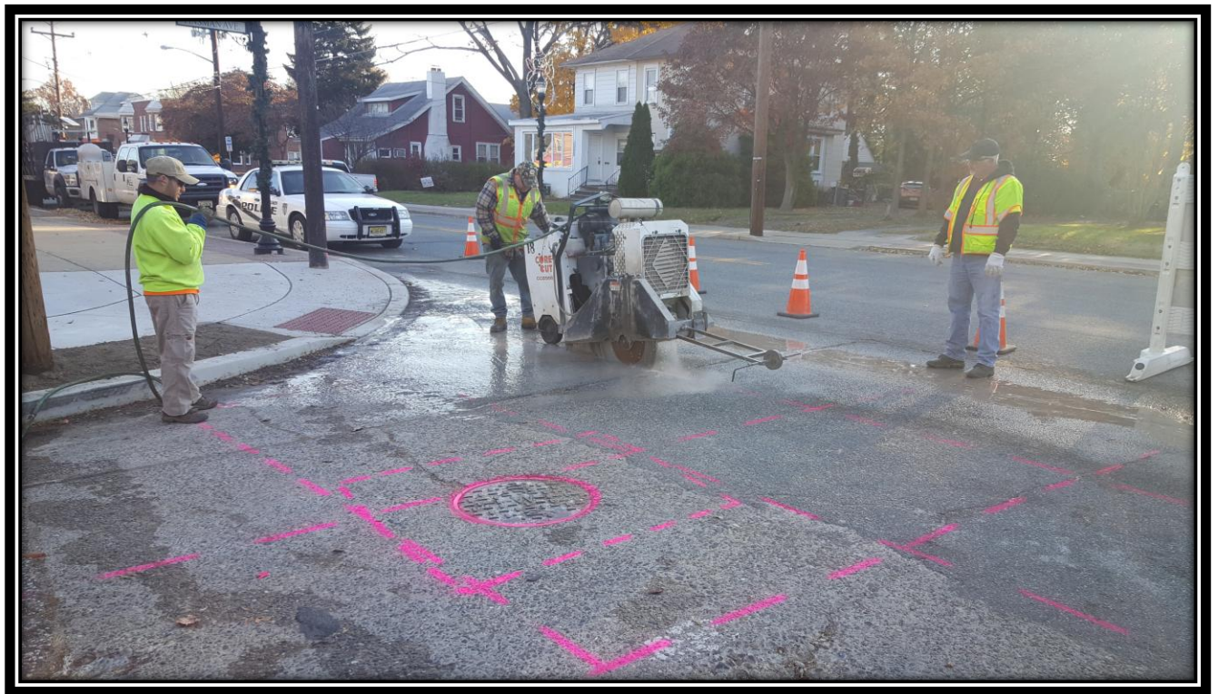
Figure: 1 – Sawcutting of existing concrete roadway to be removed at the intersection with Tinsman Avenue along the westbound lane
