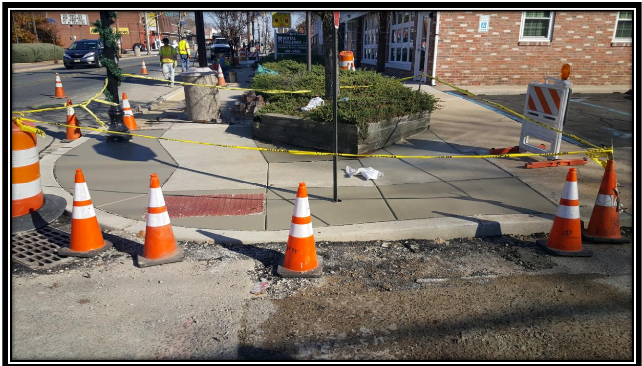
Figure: 3 – Installation of ADA ramp at the southeast corner of the intersection with 46 th Street along the eastbound lane
