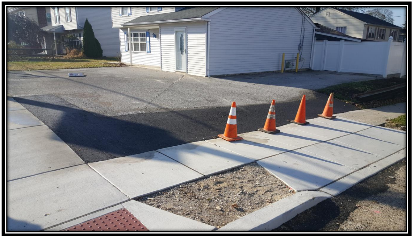
Figure: 1 – Installation of HMA driveway at the northwest corner of the intersection with 45 th Street along the westbound lane
