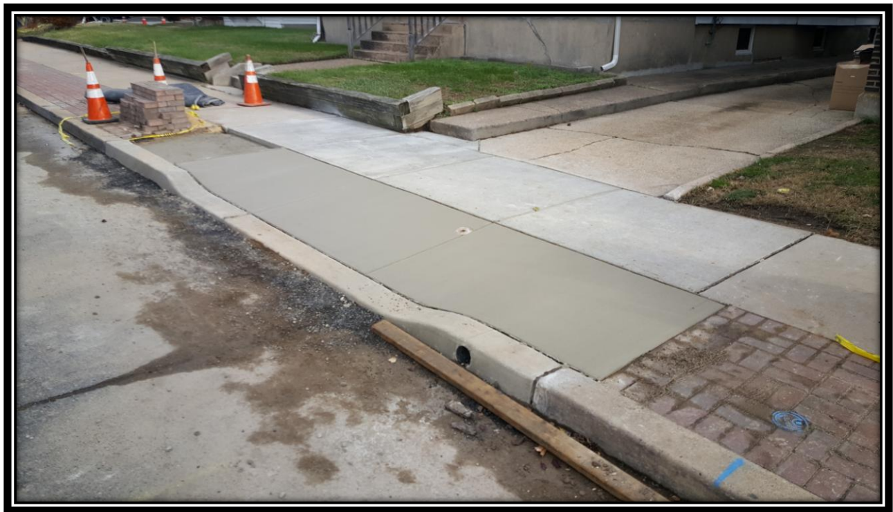
Figure: 3 – Installation of reinforced concrete driveway apron between 46 th Street and 47 th Street along the eastbound lane
