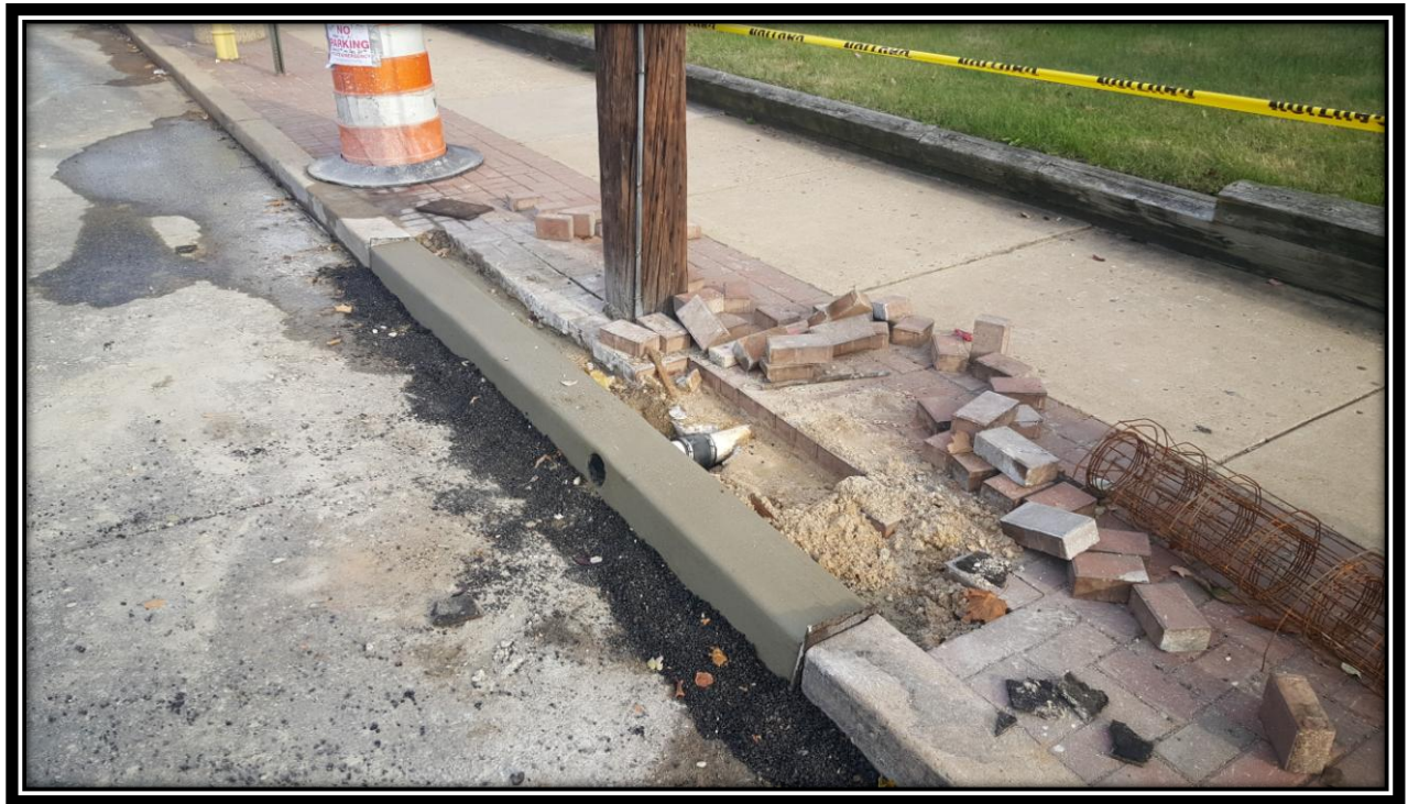
Figure: 2 – Installation of concrete curb between 46 th Street and 47 th Street along the eastbound lane
